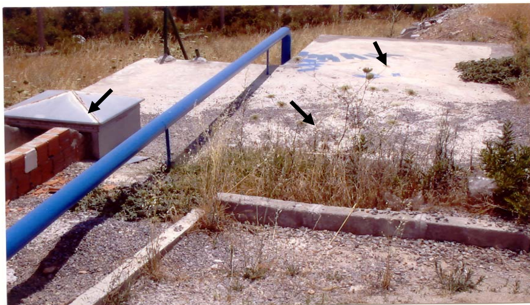
Figure 5.12: pump room at the forward, water tank at the backward and man hole of the tank.
