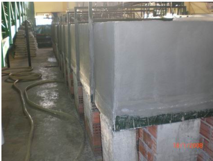
Figure A.27 Application of the insulation liquid
