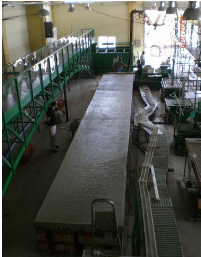
Figure A.5 Finishing of the concrete plate
