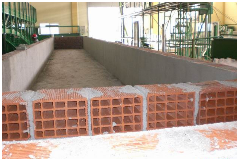
Figure A.9 Plastering of the flume
