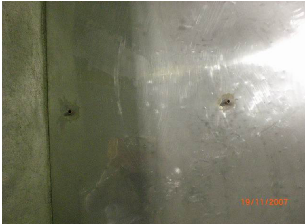
Figure A.13 The copper pipes
