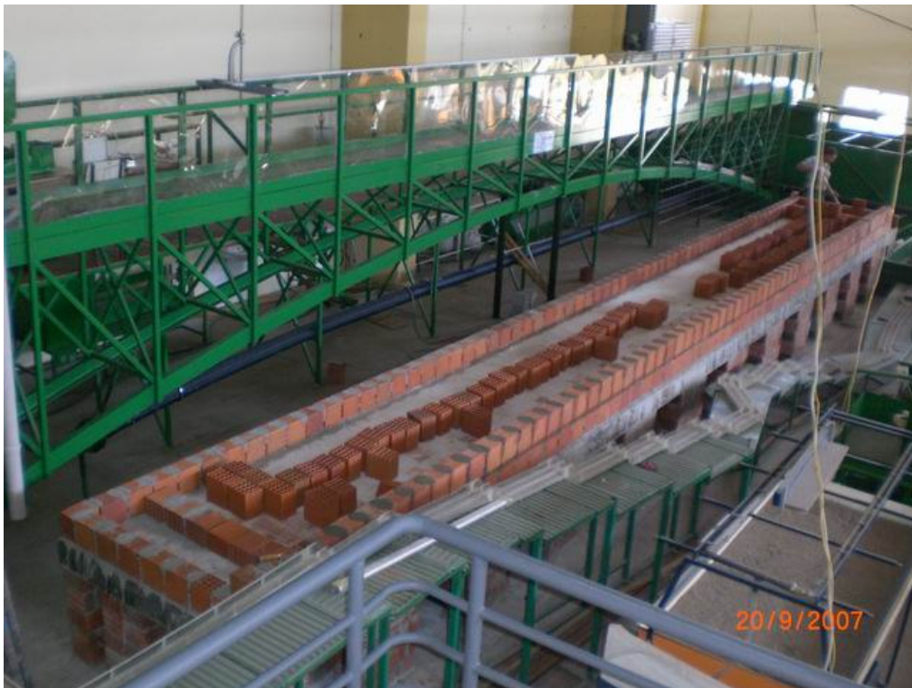
Figure A.7 Construction of the brick walls
