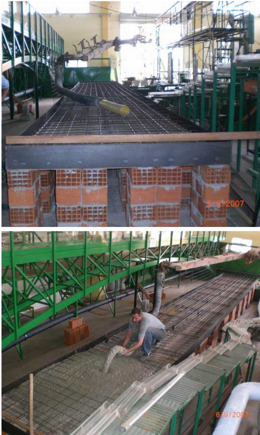
Figure A.4 Pouring of the ready-mixed concrete
