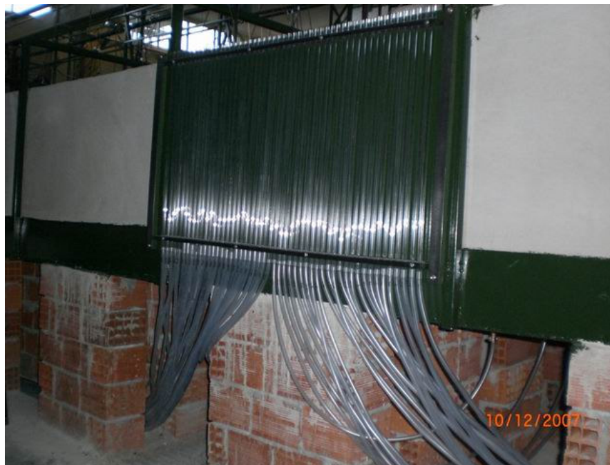
Figure 4.5 The panel of piezometers for reading the water levels
