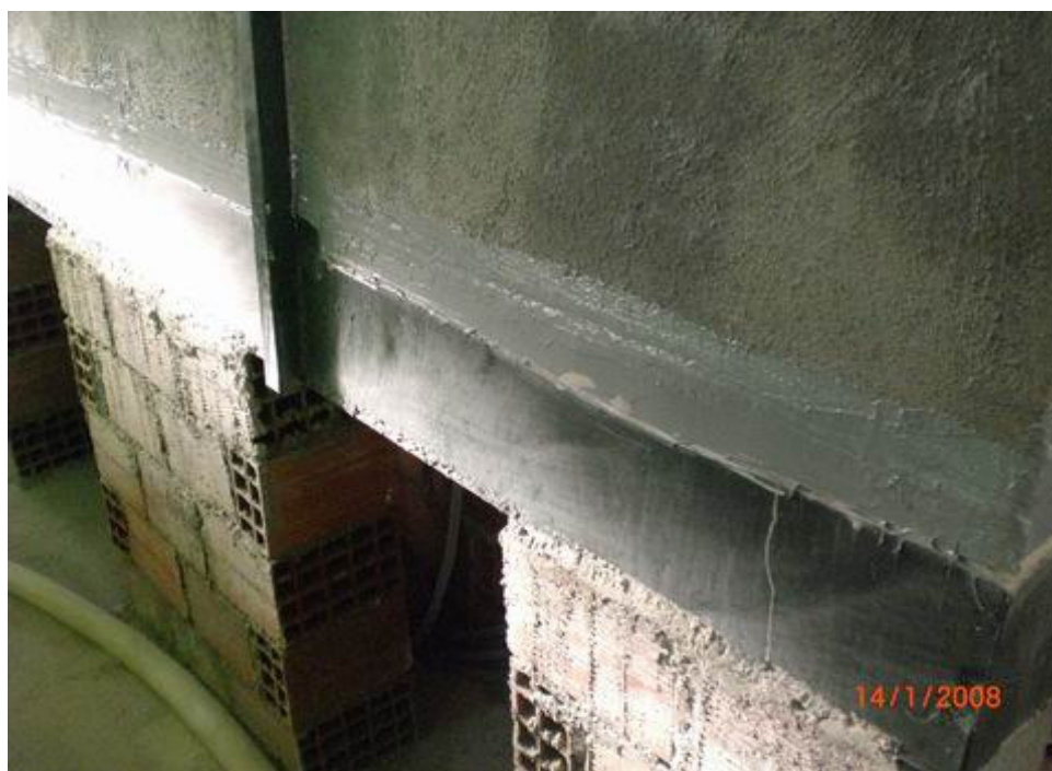
Figure A.26 Application of the insulation material
