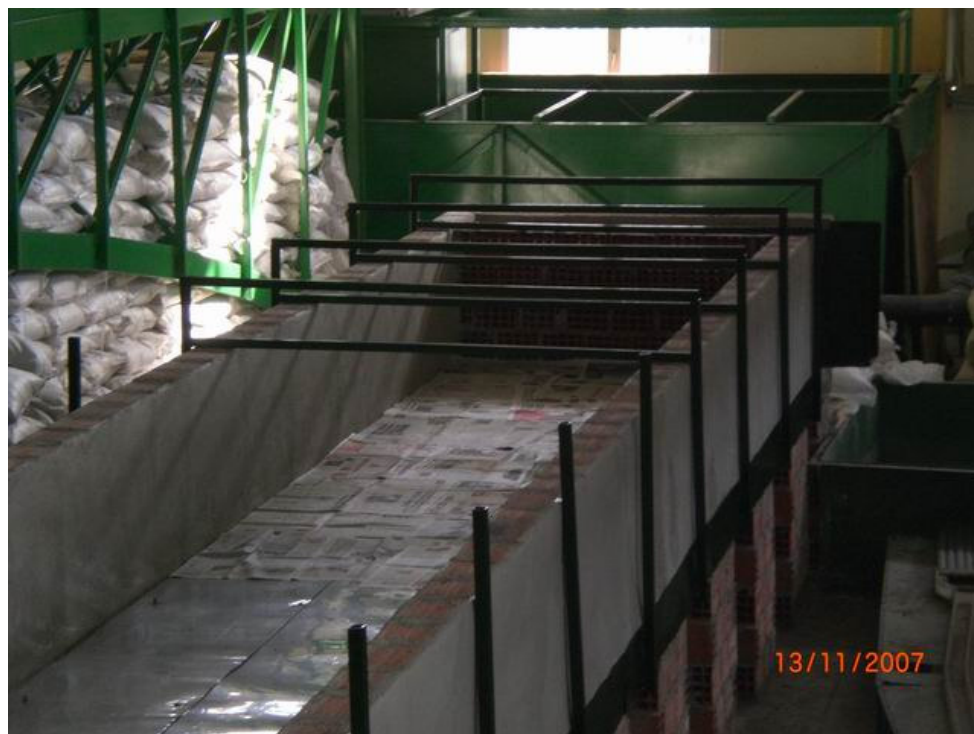
Figure A.15 Fixation of the steel profiles
