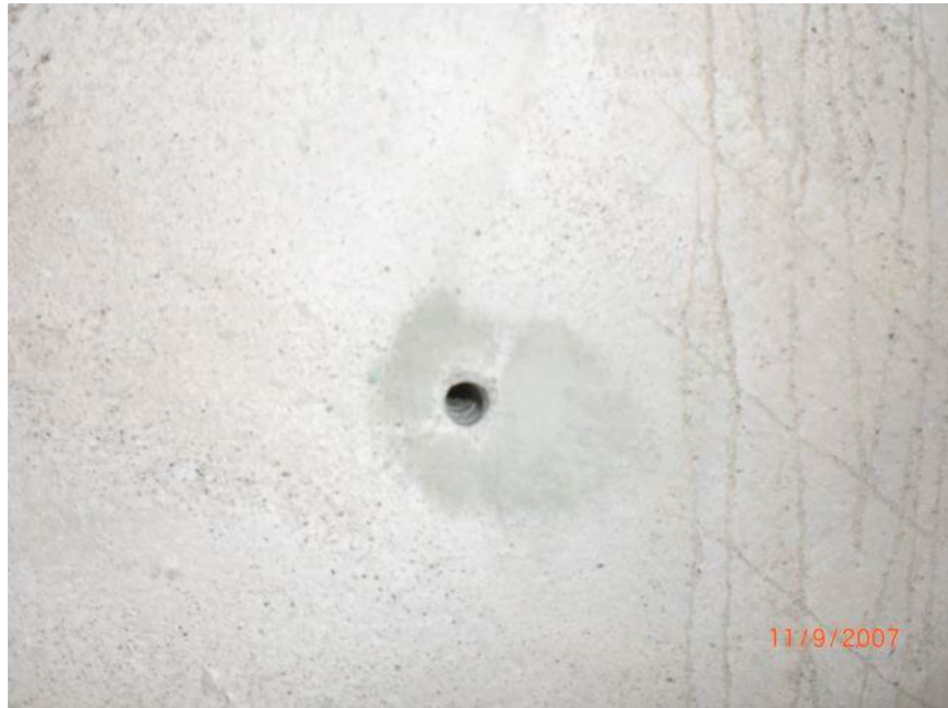
Figure A.6 The piezometer holes
