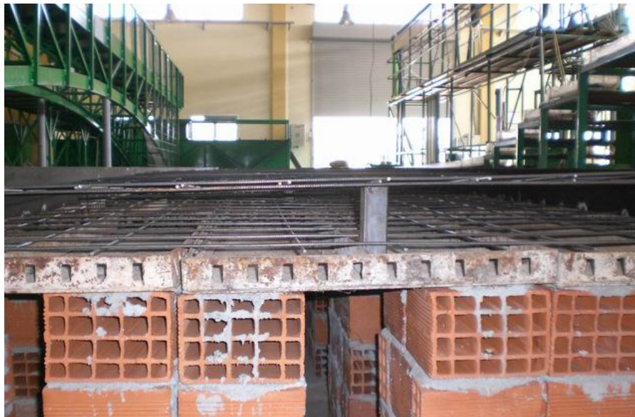
Figure A.3 Emplacement of the reinforcements
