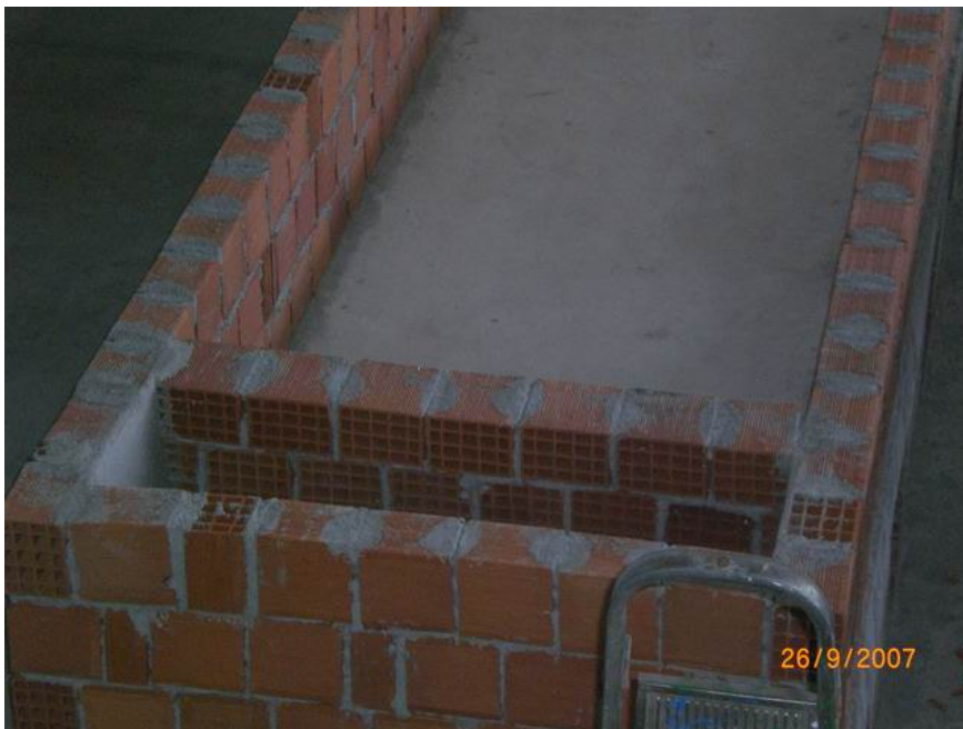
Figure A.8 The upstream reservoir and the perforated wall
