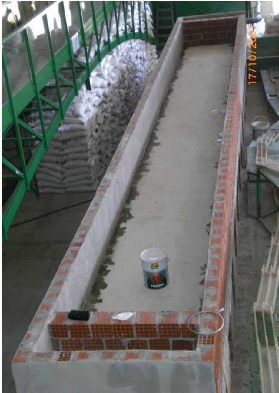
Figure A.10 Application of the water proof chemicals
