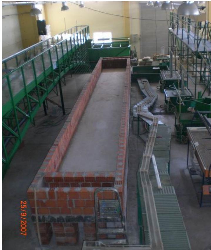
Figure A.7 Construction of the brick walls (continued)
