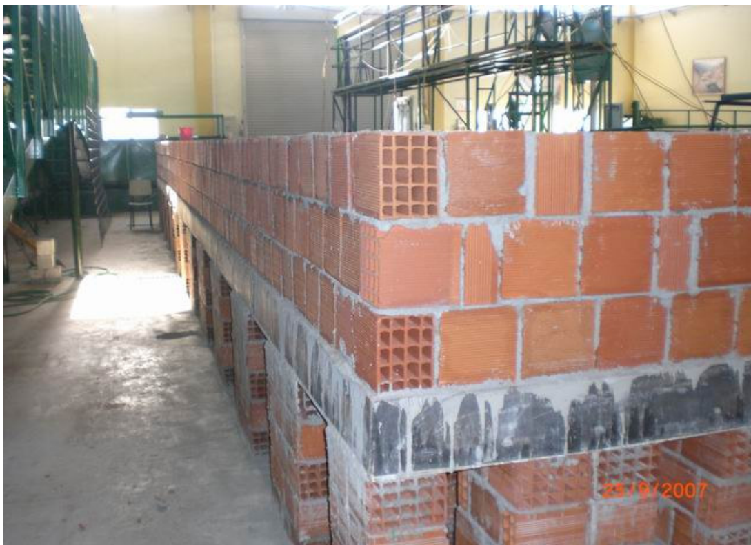
Figure A.7 Construction of the brick walls (continued)
