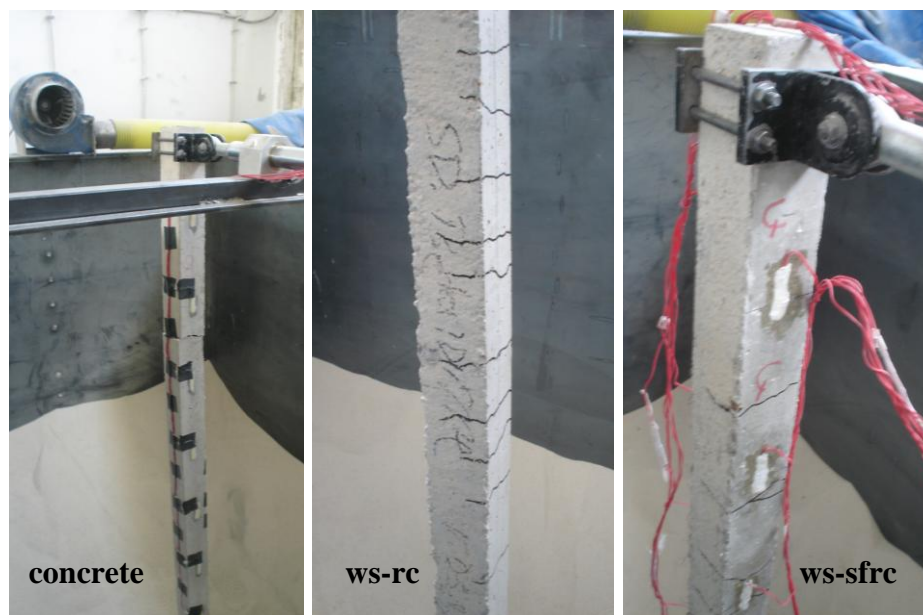
Figure 5.35 Damaged model piles after the test
