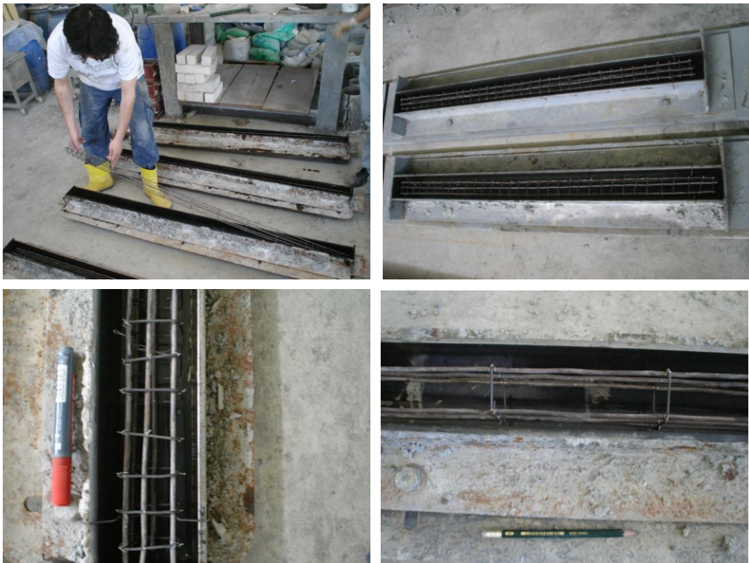
Figure 4.33 Placement of the reinforcement into the mold
