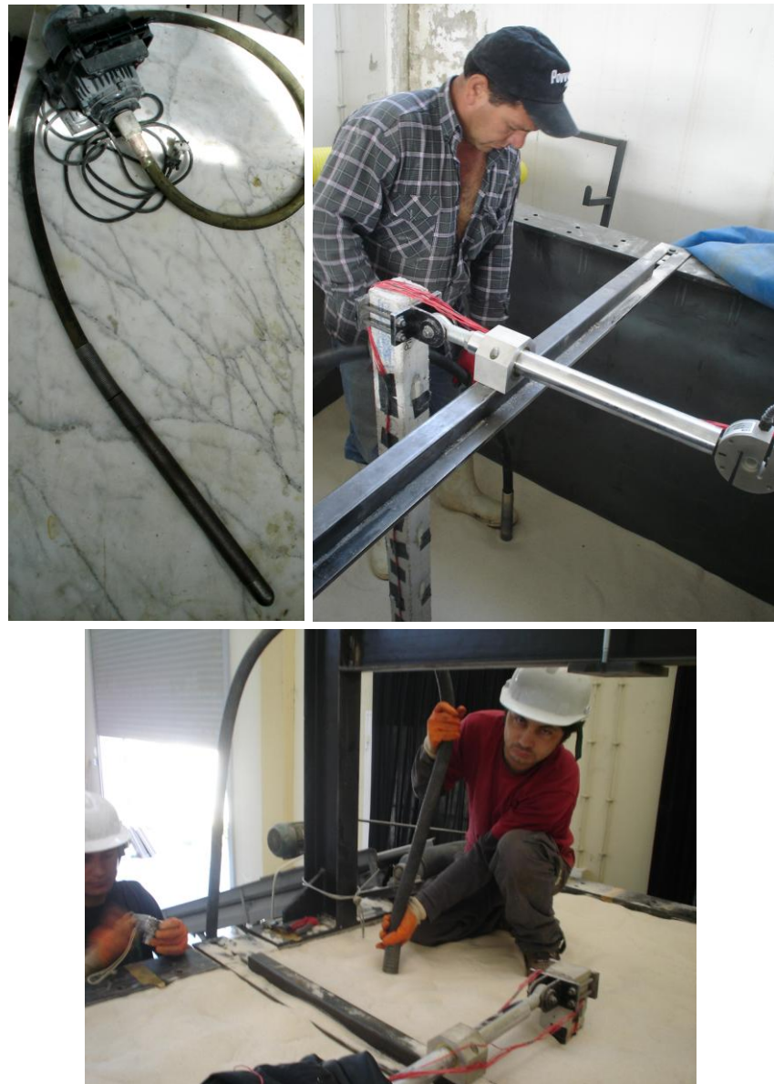
Figure 4.41 Vibratory compacter and compaction process
