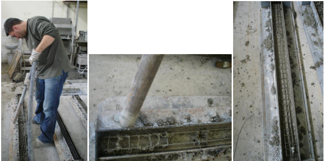
Figure 4.34 Vibration process
