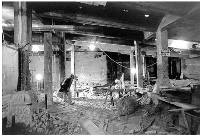
Figure 2.x Renovation process of theatre (1994) (Sherman Takata/Gensler and Associates Architects , 2009)
