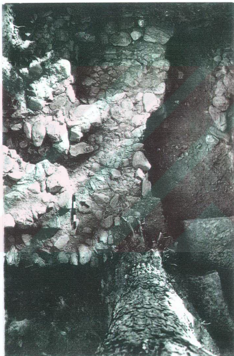
Figure 2. 11. The blockages on the east front
