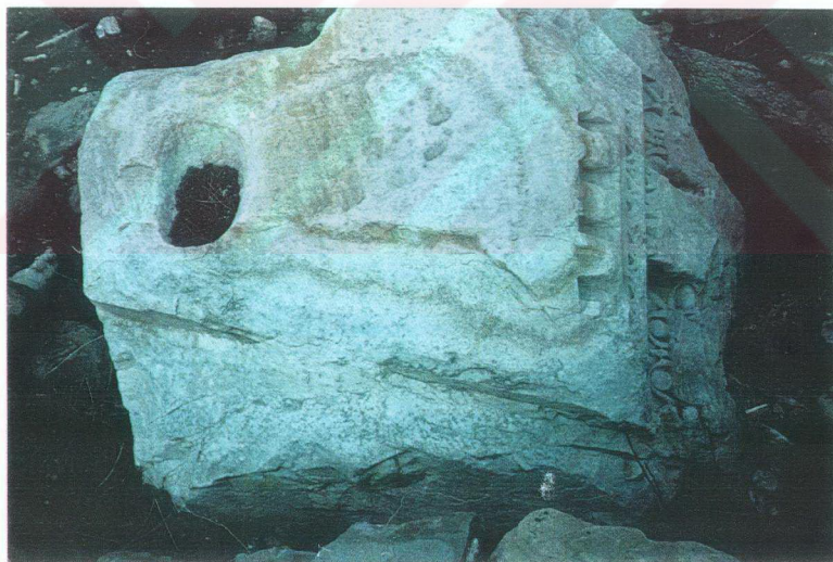
Figure 2. 35. The upper view of the cornice block ( AKR - 21 )
