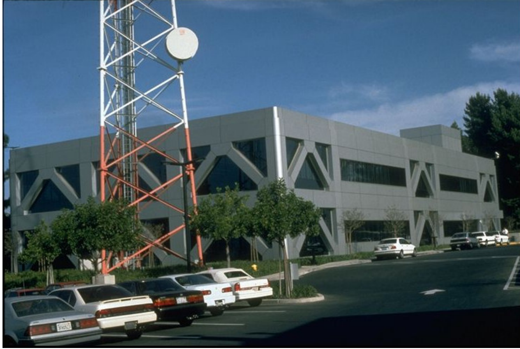
Şekil 1.4 Fire Command and Control Facility binası (University of California Berkeley, b.t.)
