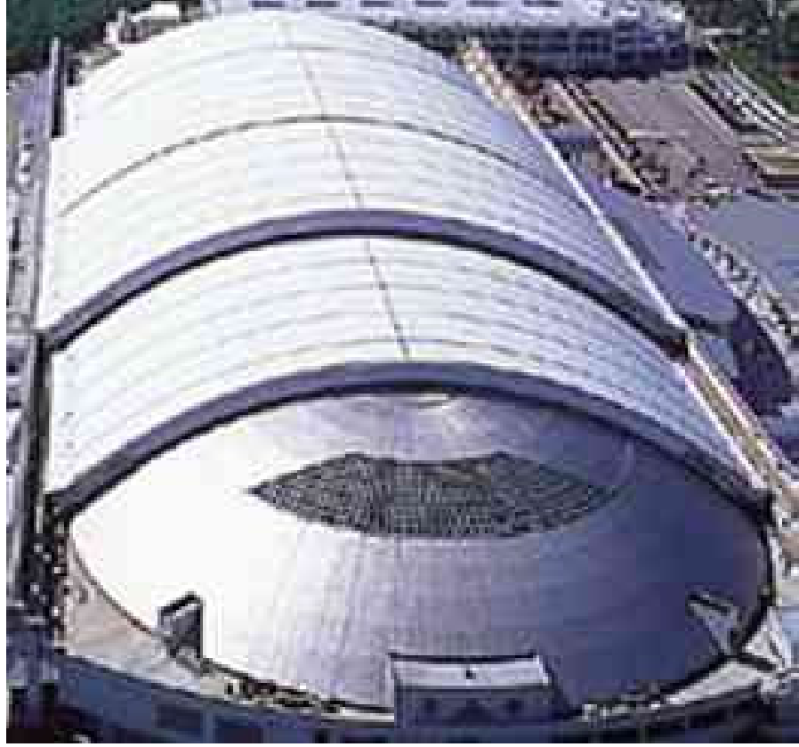
Şekil 3.105 Ocean Dome ( http://largedomes.com/largest/graphics/miyazaki_ocean_dome.jpg )
