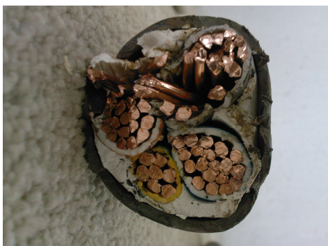
Figure 3.3 Cross section of energy cable
