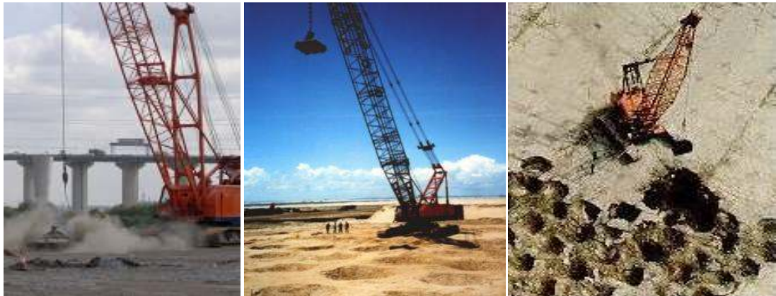
Şekil 2.3 Dinamik kompaksiyon aşamaları ( http://keller-ge.co.uk/images/cms/DynamicCompB.jpg , http://kshitiya.files.wordpress.com/2006/09/dynamiccomp.jpg , http://www.ce.washington.edu/~liquefaction/html/how/haywardpic/deepcompac.jpg ).
