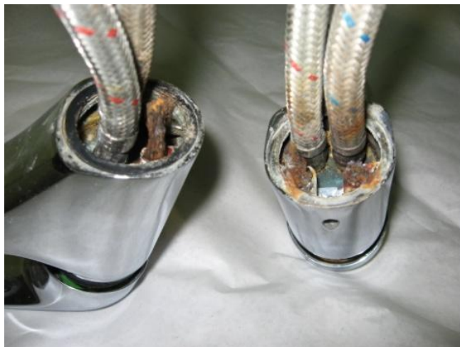
Figure 4.19 Image of two faucets with becoming rusty screws
