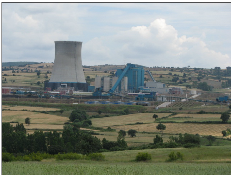
Figure 3.4 Çan Thermal Power Plant
