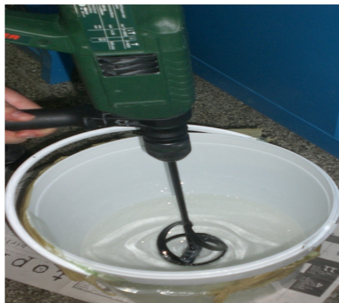
Figure 4.24 Scrambling the resin and hardener with a mixer
