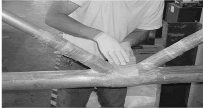
Figure 3.9 Repair of fatigue-damaged aluminum joints using glass fibre sheets ( www.civil.queensu.ca , 2009).
