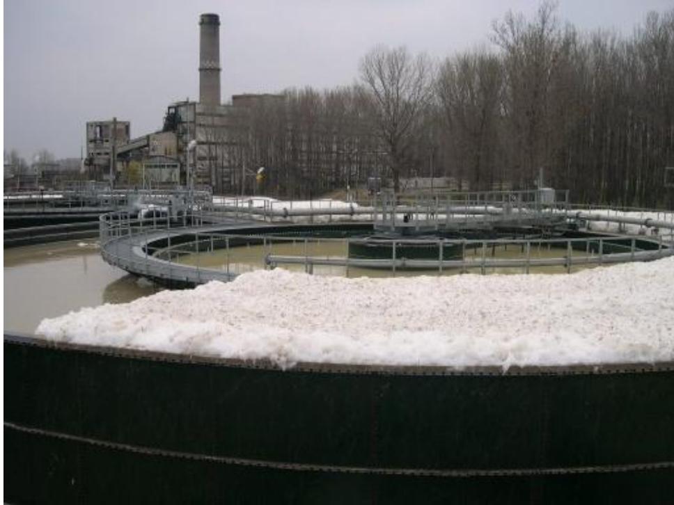
Figure 4.5 Foam Formation during start-up.
