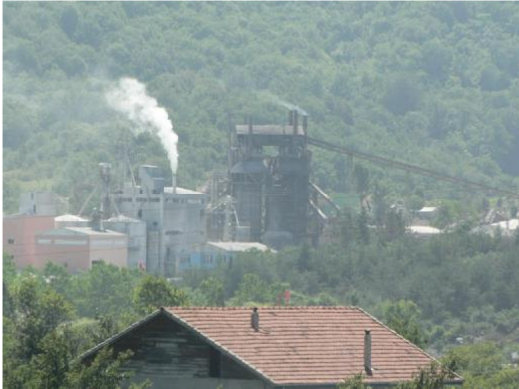
Figure: 3.2 Bartın Lime Industries.
