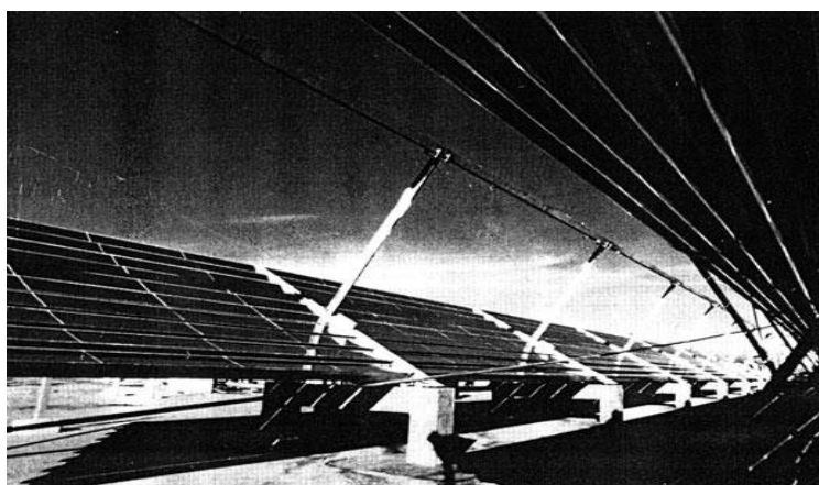
Figure 1.19 Fixed slat reflectors with tracking receiver
