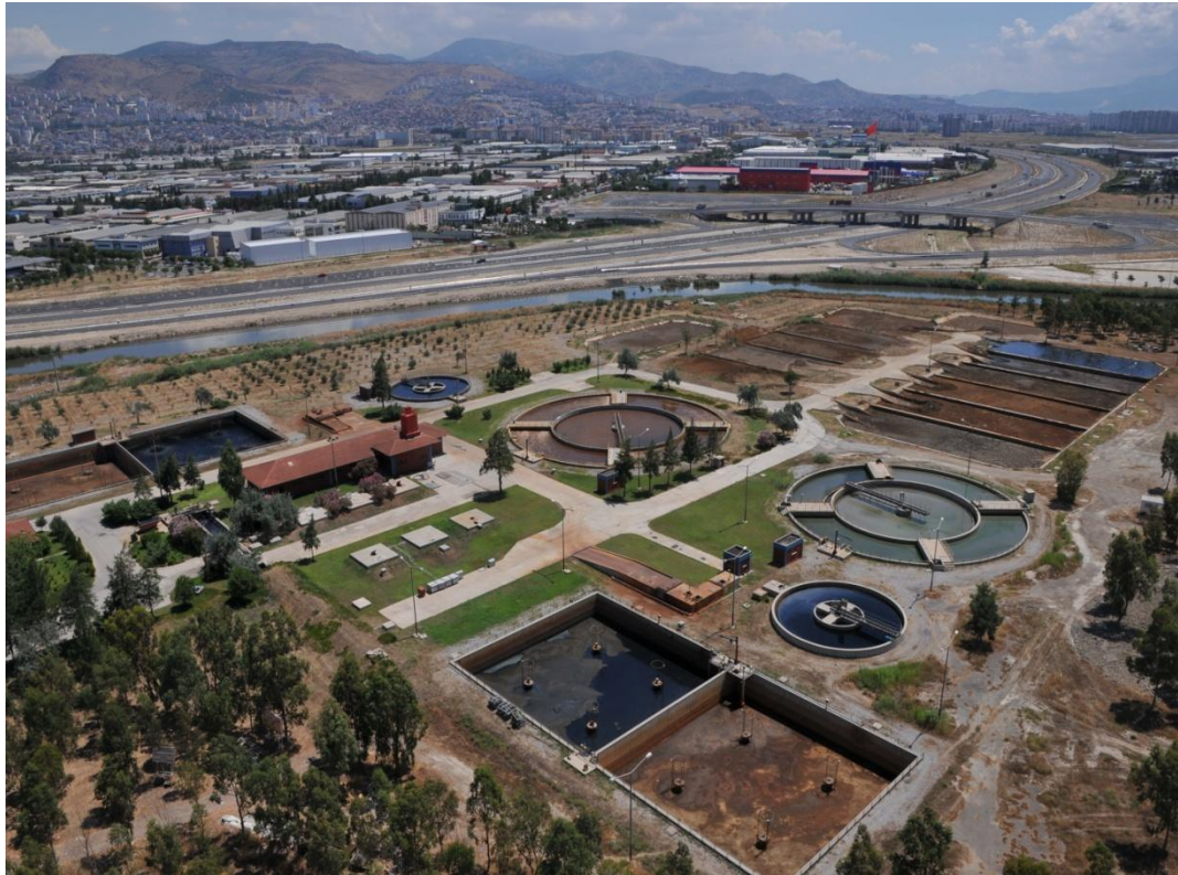
Figure 4.10 CWWTP of IAIP
