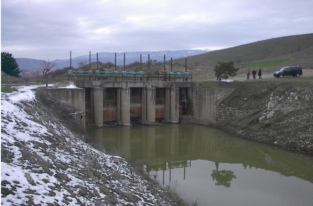
Figure. 3.3 Regulator on Simav Creek near Boğazköy
