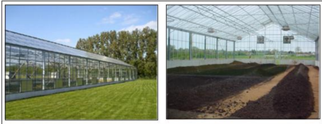
Figure 3.32 Solar sludge drying- Outside and Inside of the Greenhouse
