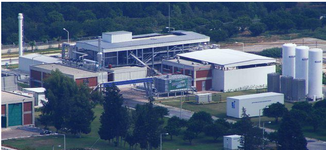
Figure 2.10 The Flow Schema of Hurma Sludge Drying Plant and a view from the plant ( www.asat.gov.tr )
