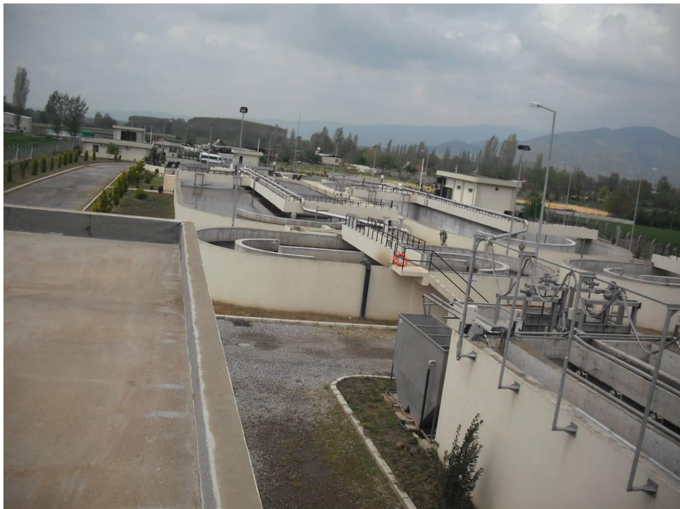
Figure 5.2 A view from Bayındır Wastewater Treatment Plant.
