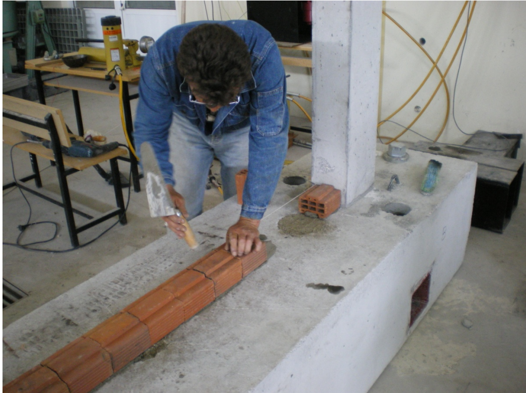
Figure 3.7 First row of locked bricks
