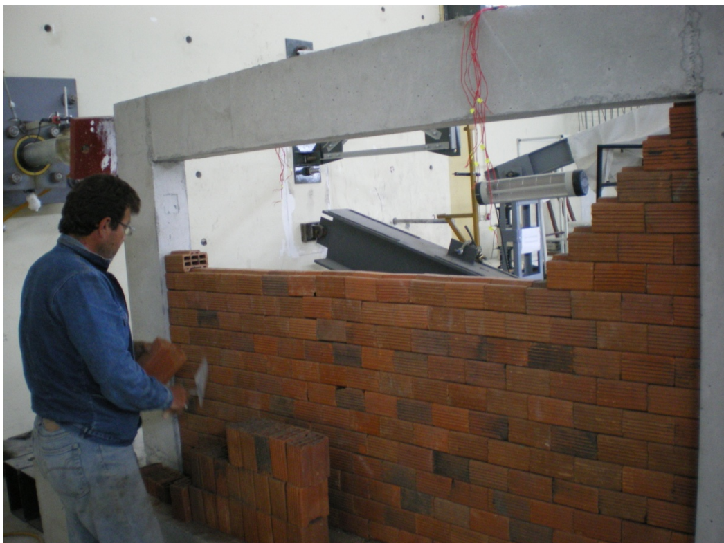
Figure 3.8 Locked brick usage during construction
