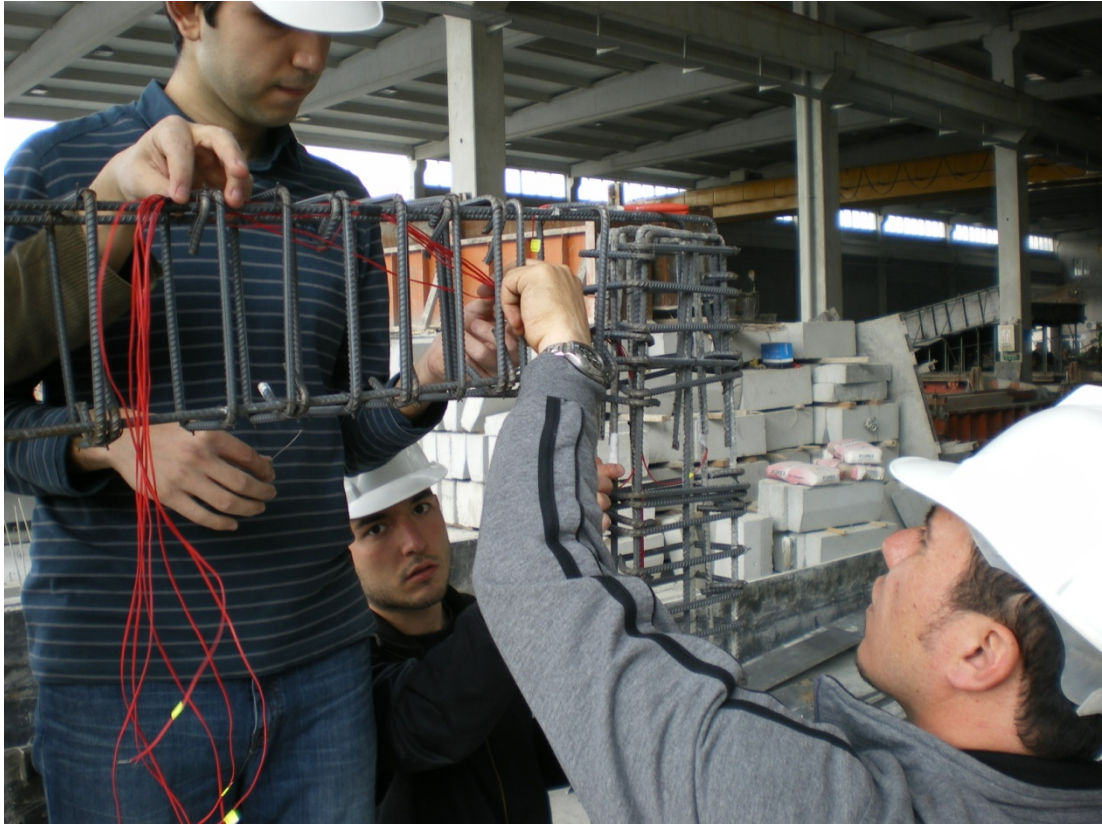
Figure 3.22 Forming of connecting cables
