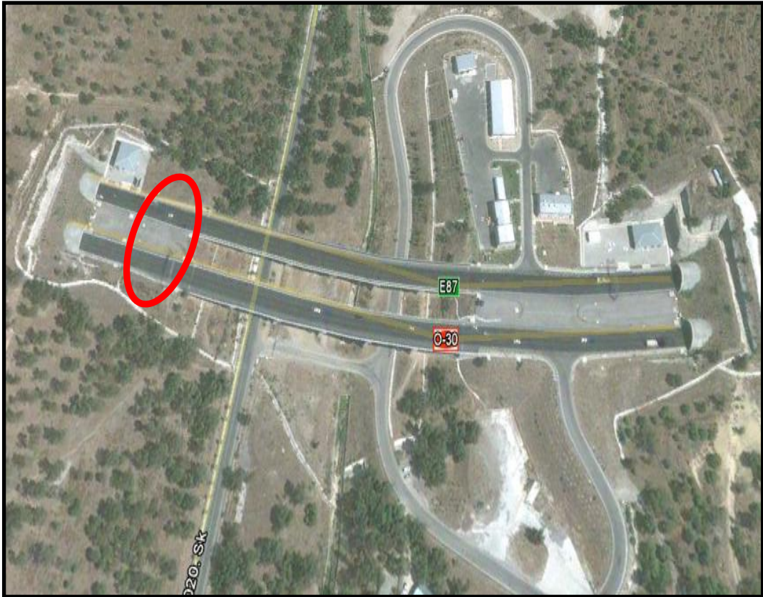
Figure 2.4 Observation site IV: Karşıyaka Tunnel
