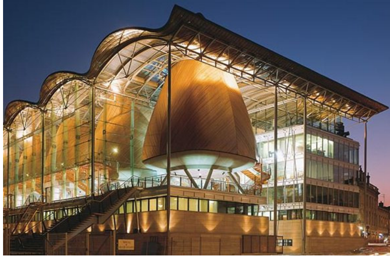
Şekil 2.19 TGI Binası, Bordeaux (Fransa) ( http://www.richardrogers.co.uk/work/all_projects/bordeaux_law_courts/completed ).
