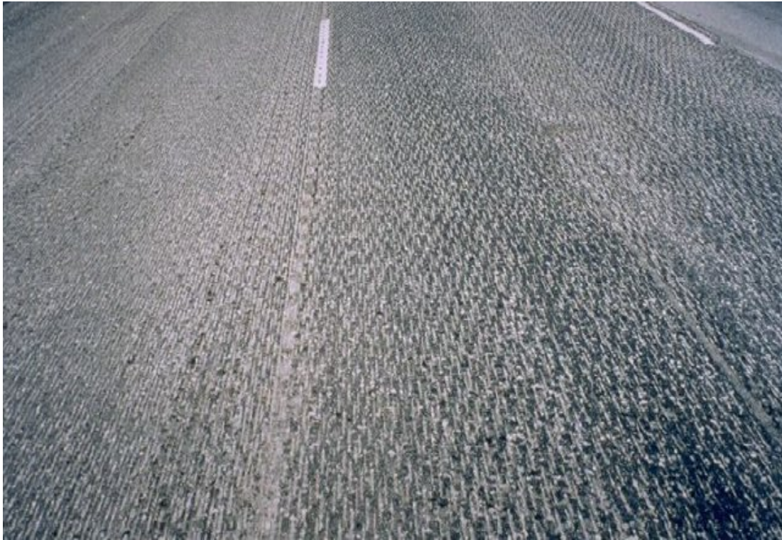
Figure 2.1 A typical surface resulting from cold milling.
