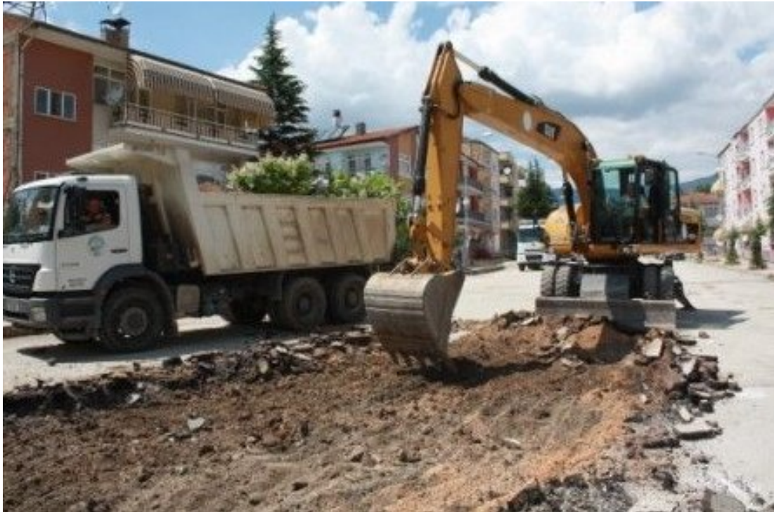
Figure 2.2 A typical surface resulting from ripping and crushing.
