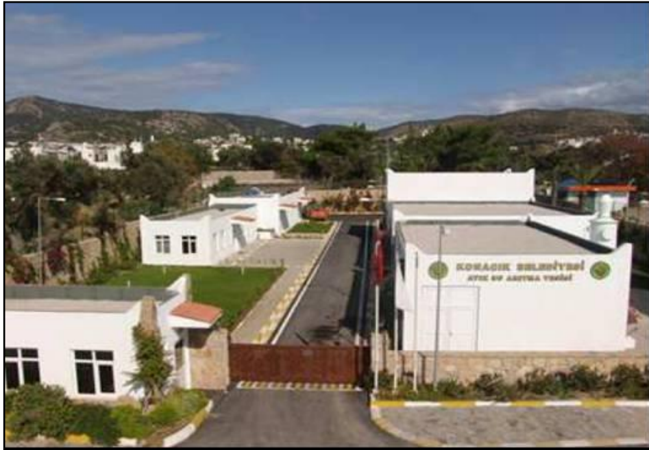
Figure 3.1 General view of Konacık wastewater treatment plant
