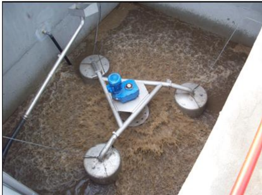
Figure 3.14 Thickening tank
