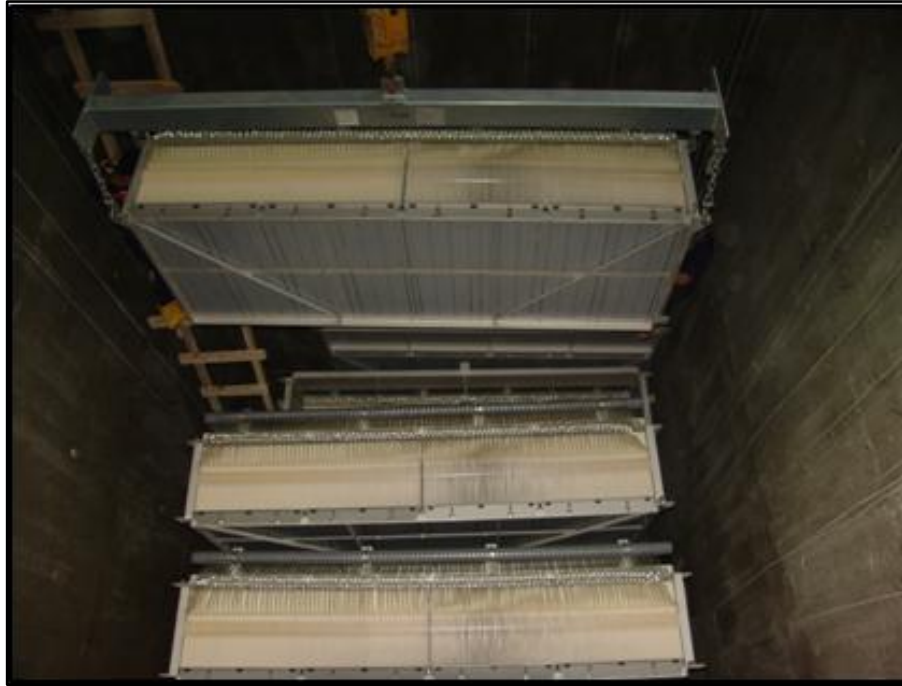
Figure 3.11 MBR installation
