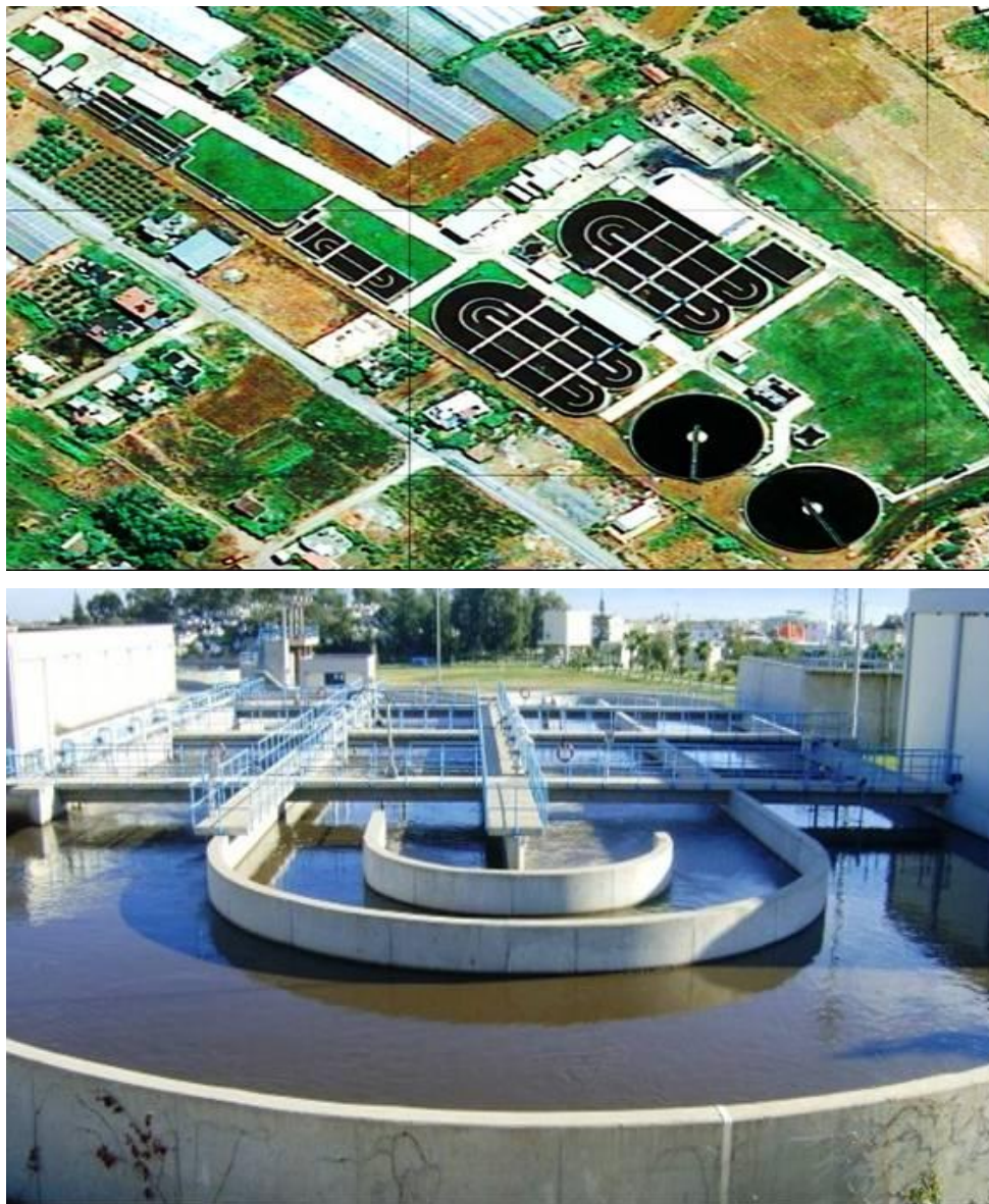
Figure 5.4 Fethiye wastewater treatment plant, Muğla/Türkiye
