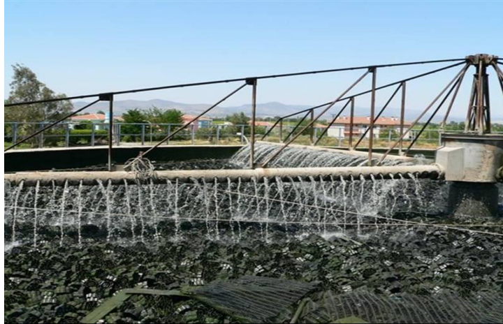
(a) Trickling filter
