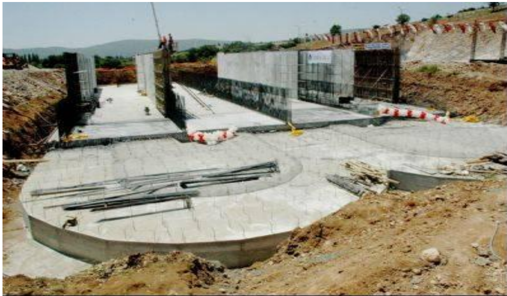
Figure 5.17 The construction of the Mugla municipal wastewater treatment plant.
