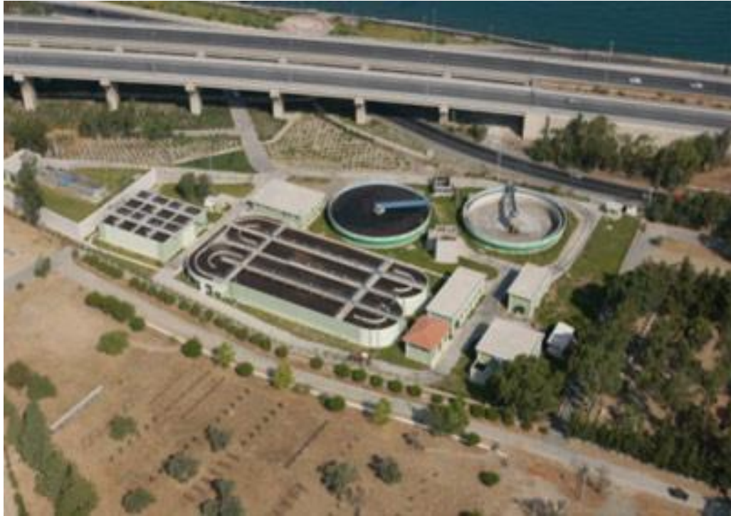
Figure 5.2 Güneybatı wastewater treatment plant, İzmir/Türkiye
