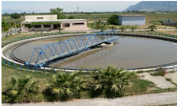
(a) Sedimentation Tank
