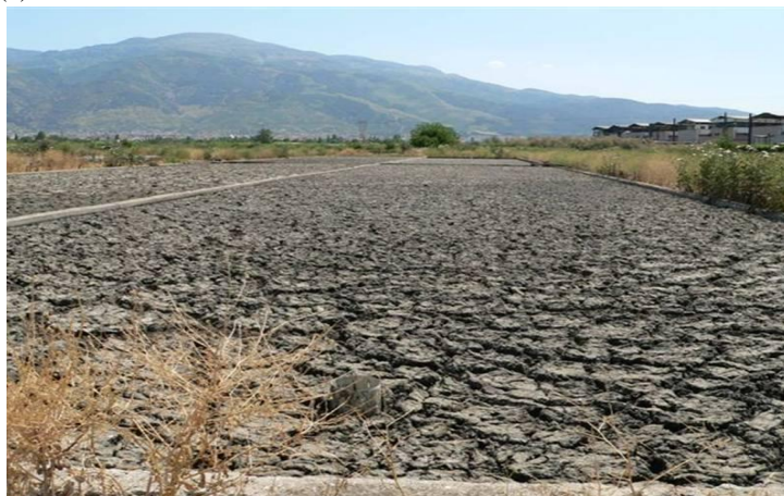
(c) Sludge drying beds
