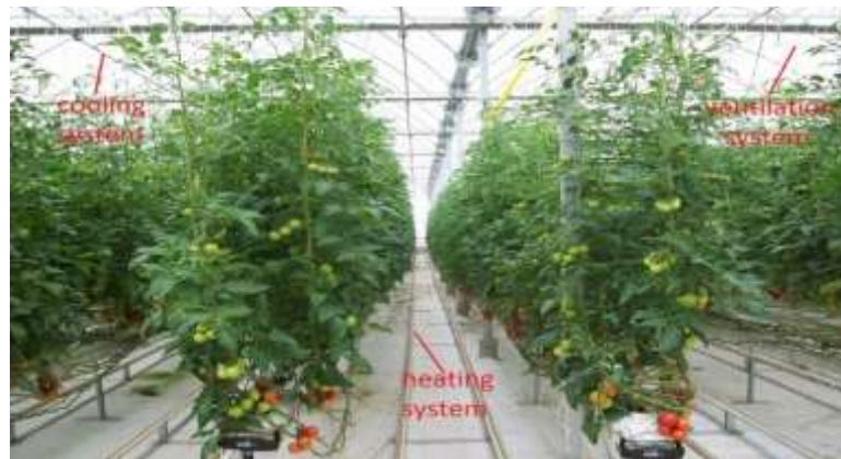
Figure 1.3 Systems in Greenhouse
