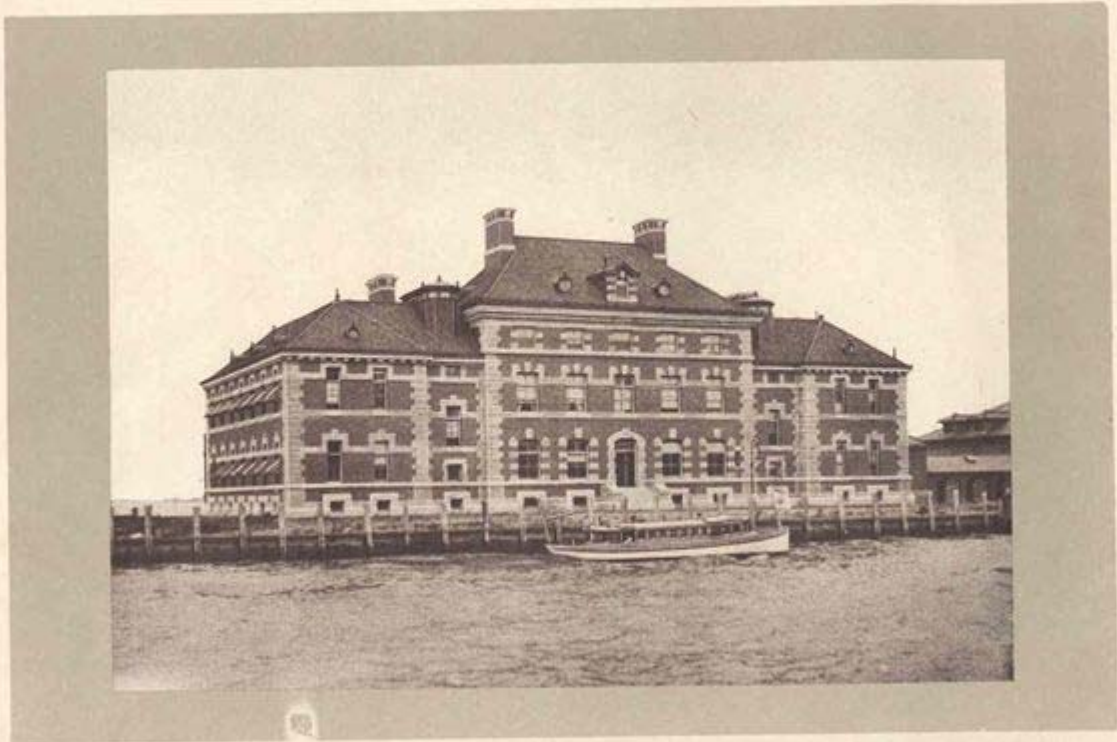
NEW HOSPITAL BUILDING, ELLIS ISLAND.
