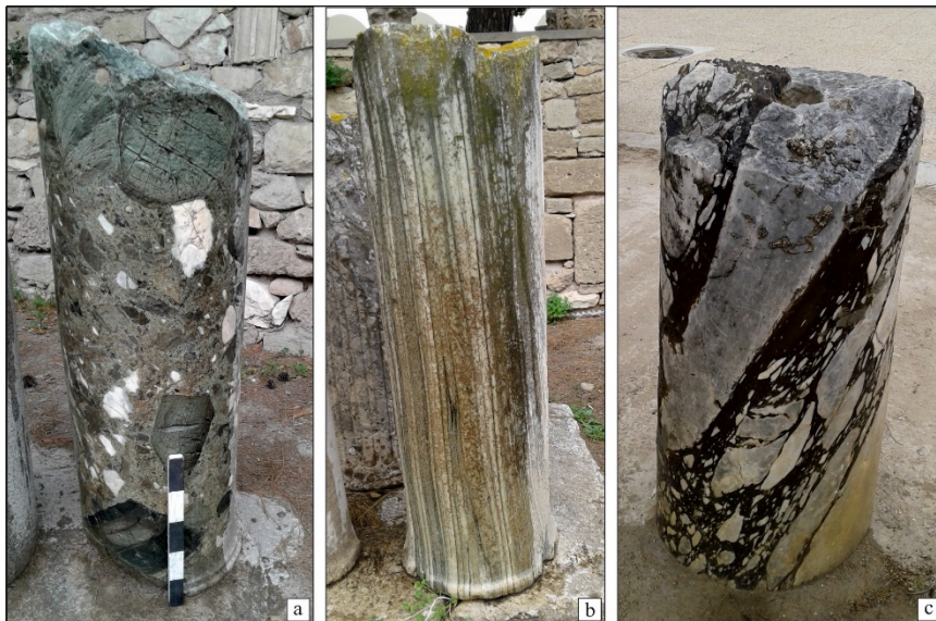
Figure 6: Fragmentary column shafts of Greek coloured marbles: a. smooth verde antico; b. smooth cipollino verde; c. smooth breccia di Settebasi.
