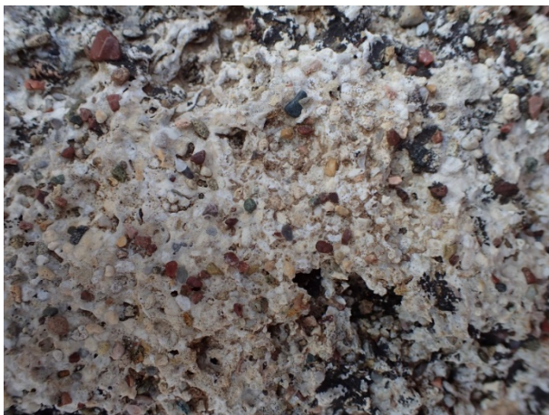
Figure 7: Close-up view of calcareous sandstone from the krepis of the Nike Monument in the Sanctuary of the Great Gods. (field of view 60 mm). Note variety of clasts consisting of basalt, jasper, fossils, limestone, quartz, and rhyolite (Photo: Authors).
