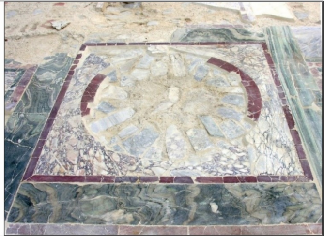
Figure 3: Detail of the floor showing the emblema in the center of the room with cornices of cipollino verde and rosso antico contouring a fragmented roundel of proconnesian marble and a breccia di settebasi infill (Photo: E. Gallochio).
