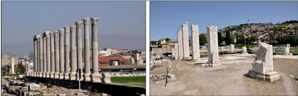
Figure 4: Smyrna, Agora, western stoa. View from southwest of the outer colonnade replaced in the fifties of the 20th century. Troad and Kozak granites are used for the shafts (Photo: M. Bruno). Figure 5: Smyrna, Agora. Overview of the central nave of the Basilica with pillars in red breccia from Manisa (Photo: M. Bruno).
