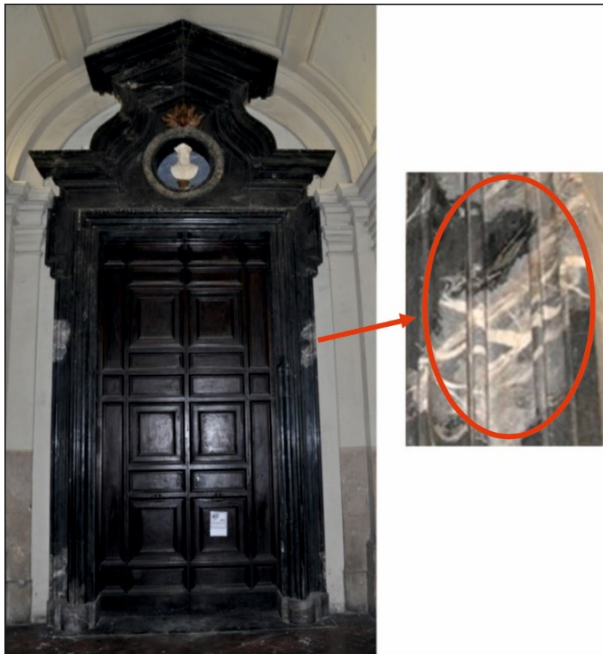
Figure 5: The large door leading to the main Oratorio room with a detail of the yellowish inclusions visible in various parts of the Göktepe black marble jambs (Photo: D. Attanasio).
