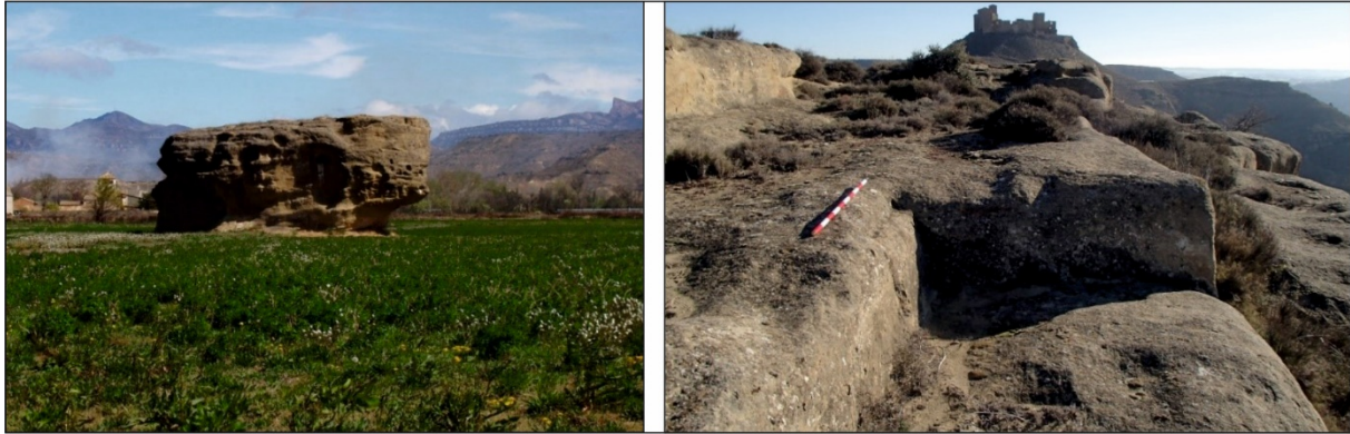
Figure 9: An old sandstone quarry near Huesca. Most of it has been repurposed as an agricultural field. The rest of the rock was probably used during the Islamic period as the foundations for a watchtower (Photo: J.A. Cuchí).
