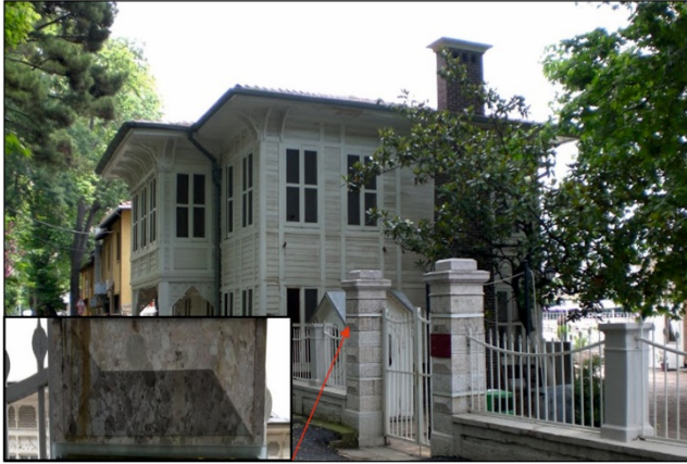
Figure 1: Hereke puddingstone on the garden walls of Kaiser Wilhelm Mansion in Hereke.
