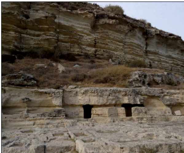
Figure 7: Detail of the layering of the cliff in area B where the upper yellow layer consists of chalky marls, very weathered, and the lower one relates to the hard grey limestone of the chamber tombs and quarry floor (Photo: M. Astolfi).
