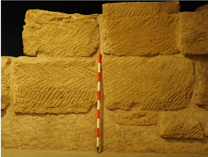
Figure 1: Roman ashlars in the basement of the administrative headquarters of the Province of Huesca (Photo: J.A. Cuchi).
