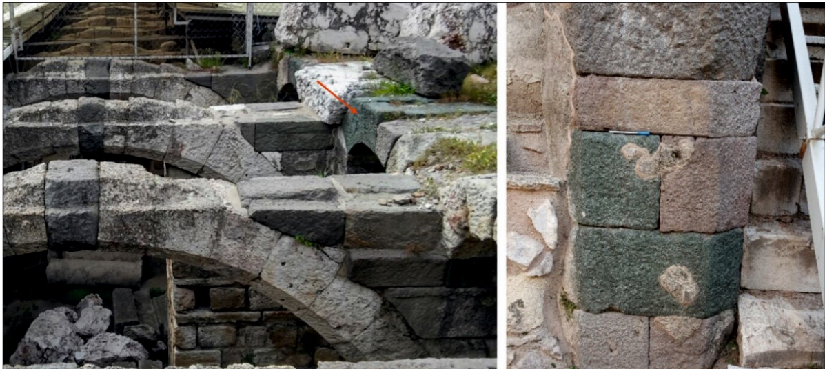
Figure 2: Green stones used in the arch structures and in the wall blocks in the Smyrna Basilica basement, pen size is 16.5 cm (Photo: B. Yolaçan).
