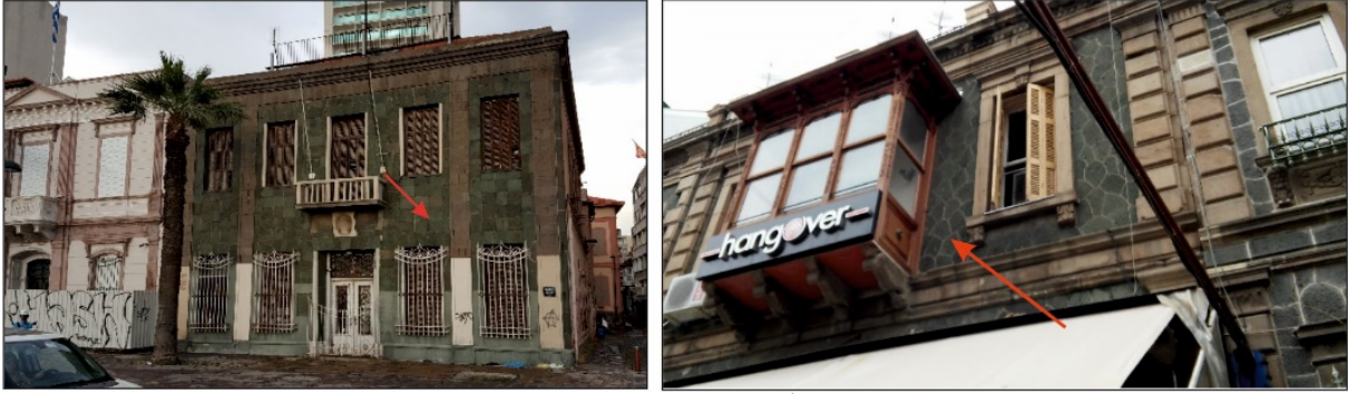
Figure 3: Green rock used in the historical buildings in Alsancak-İzmir (Photo: M Çolak).
