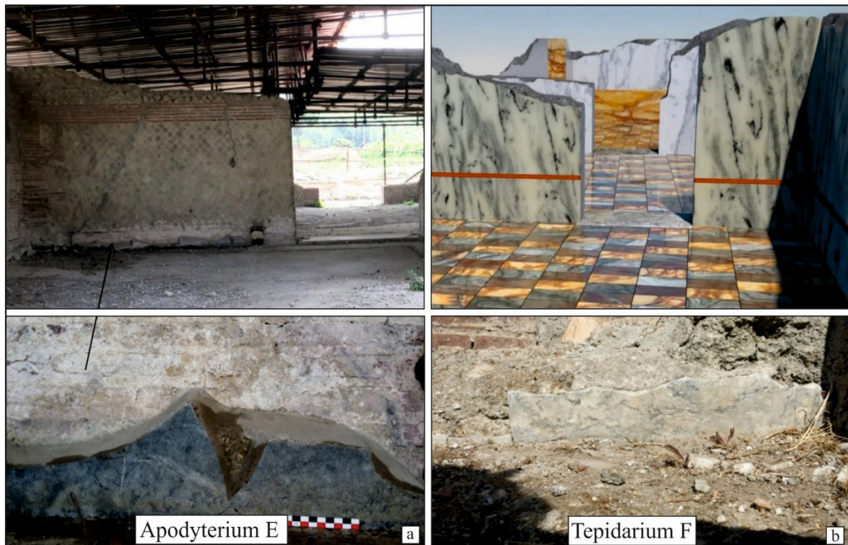
Figure 10: Greco scritto at Cumae (Cuma). Details of marble remnants: a. room E; b. room F with 3D reconstruction (Photo: R. Scognamiglio, 2016).
