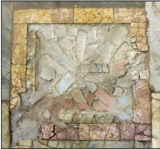
Figure 2: An example of a portion of the floor still retaining the potsherd amphora-fragments used to fix the various marbles in a panel, and the imprint of the latter attesting the prefabrication of the opus sectile elements (Photo: E. Gallochio).
