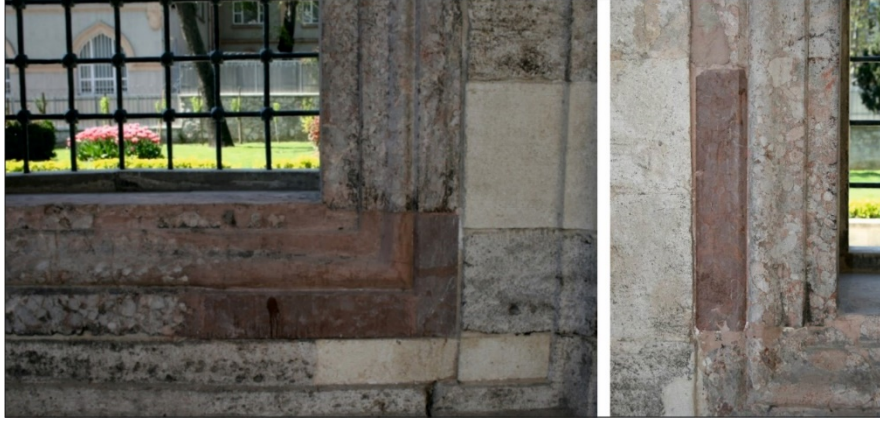
Figure 16: Examples of imitation stone applications used instead of the Hereke puddingstone in the frames of courtyard windows in the restoration of Yavuz Selim Mosque (dark colored parts are covered with imitation materials made of pigmented mortar).
