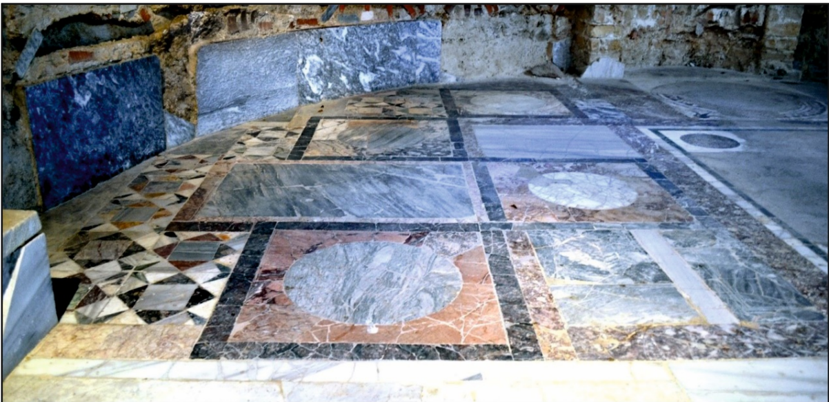
Figure 4: Detail of the apse's floor showing a large use of bardiglio and portasanta (Photo: S. Prestifilippo).
