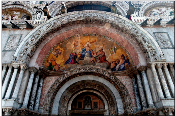
Figure 4: Hereke puddingstone used as lateral pediment cladding on the main arched gate of St. Mark's Basilica in Venice, Italy.
