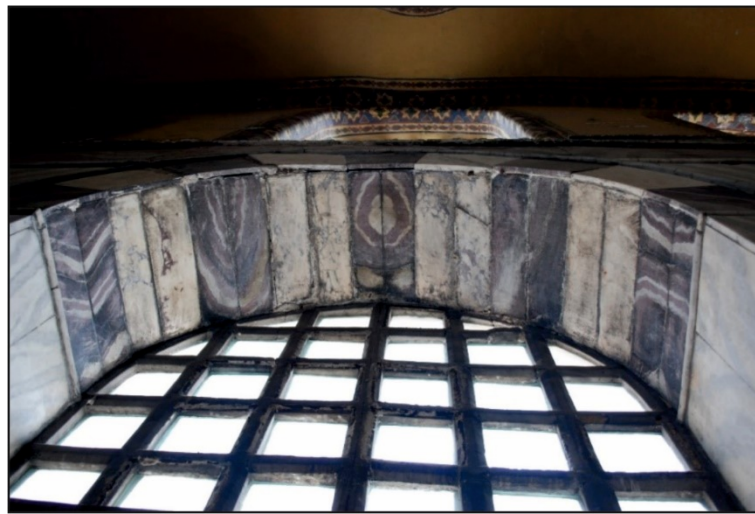
Figure 10: Istanbul, Hagia Sophia: the intrados of a windows galleries arc alternating red cipollino and pavonazzetto (Photo: D. Peirano).
