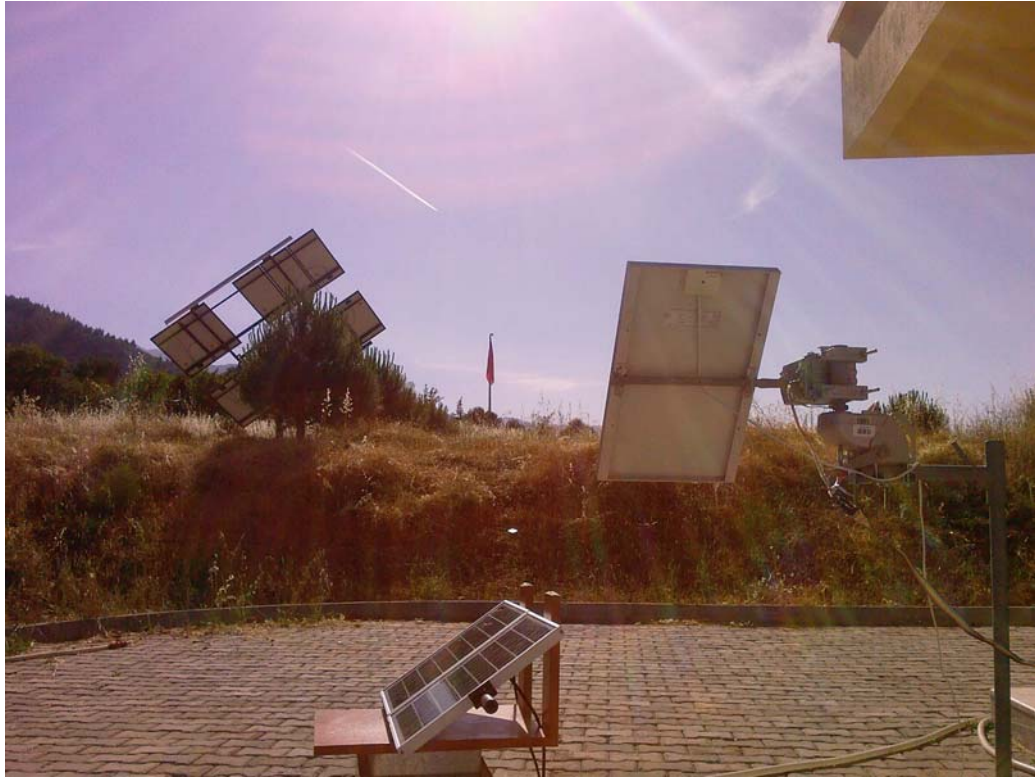
Figure 4.30 A view from the work where two-axis tracking system are compared with a fixed system.
