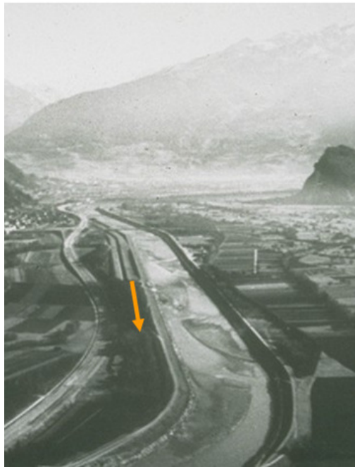
Figure 4.14 The alternate bars in Rhine River, Lichtenstein, Switzerland (Parker, 2006)
