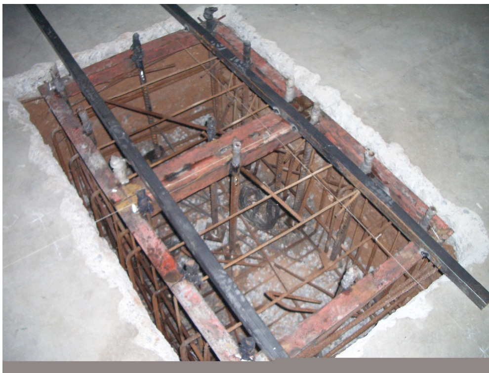
Figure A.13 The footing of the flume supports
