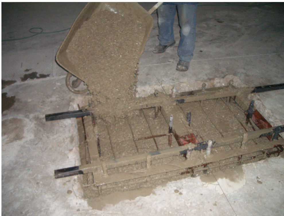
Figure A.14 The footing of the flume supports
