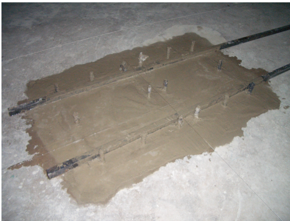
Figure A.15 The footing of the flume supports
