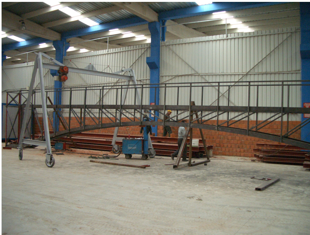
Figure A.18 Construction of the skeleton of the channel
