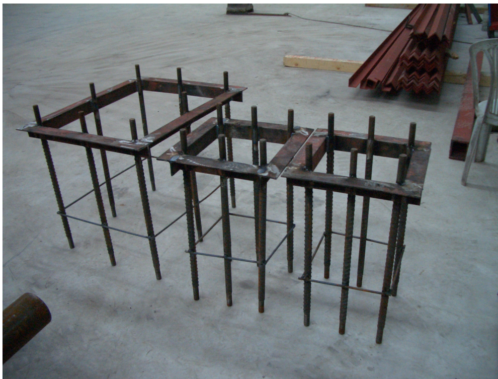
Figure A.12 The footing of the flume supports
