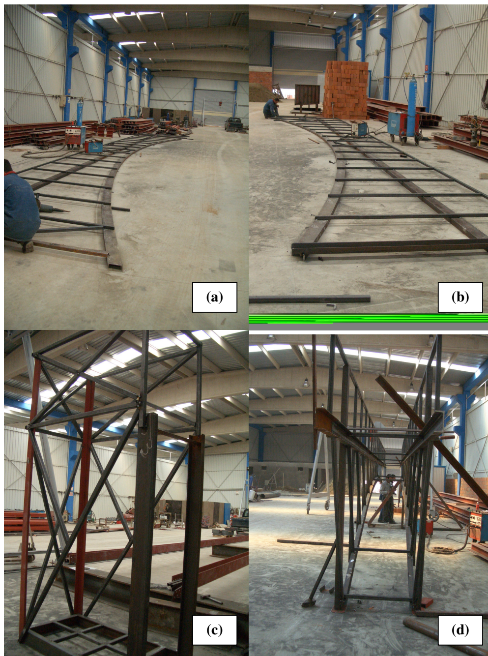
Figure A.16.a,b,c,d Construction of the skeleton of the channel
