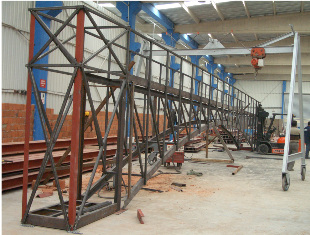
Figure A.17 Construction of the skeleton of the channel
