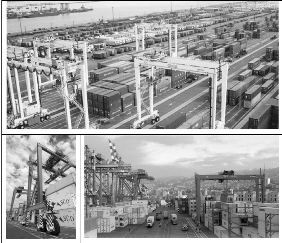
Figure 5.42 Unmanned gantry cranes (RTGs) at yard area. Source: Kalmar industries 2009
