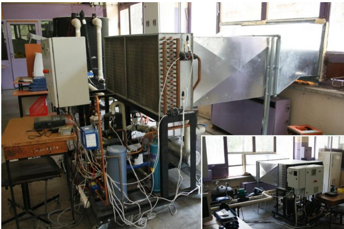
(b) Chiller and components
