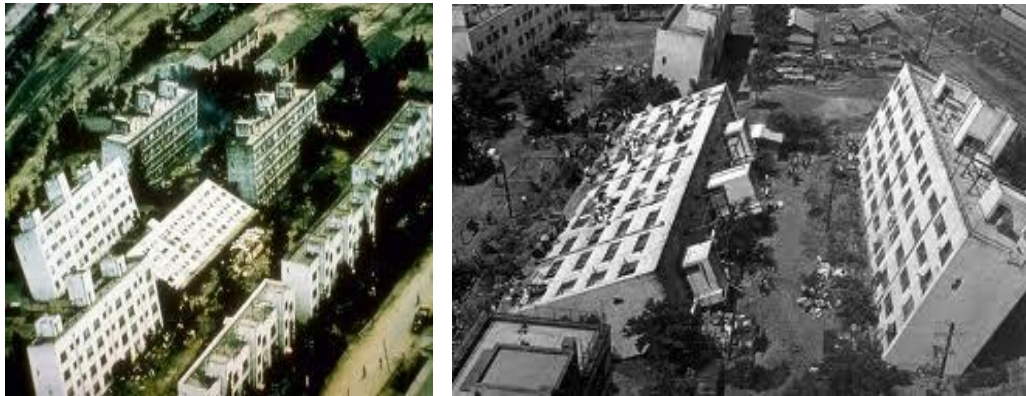
Figure 2.3 The loss of bearing capacity of foundation due to liquefaction in 1964 Niigata Earthquake ( http://www.architectureweek.com/2012/0307/ , 2012; Photos by Youd T.L., 1964)
