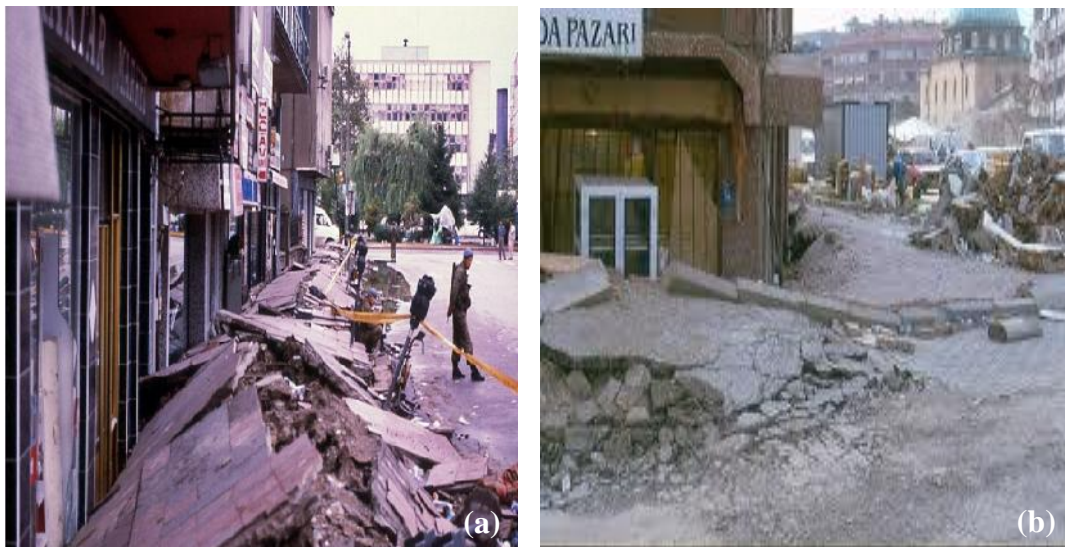
Figure 2.2 Liquefaction traces and post liquefaction excessive settlement in Adapazarı city center in 1999 Marmara Earthquake (a: http://sezayozbal.blogspot.com/2011/11/99-depremi-golcuk-adapazar-8.html , 2011; photo: Özbal S., 1999; b: http://kisi.deu.edu.tr/huseyin.catal/ , 2011; photo: Çatal H.H., 1999)
