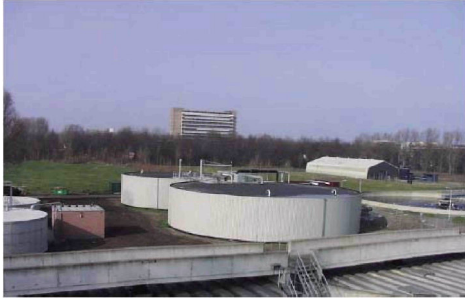
Figure 2.15 The SHARON plant in Utrecht (Grontmij Water & Reststoffen, 2004)
