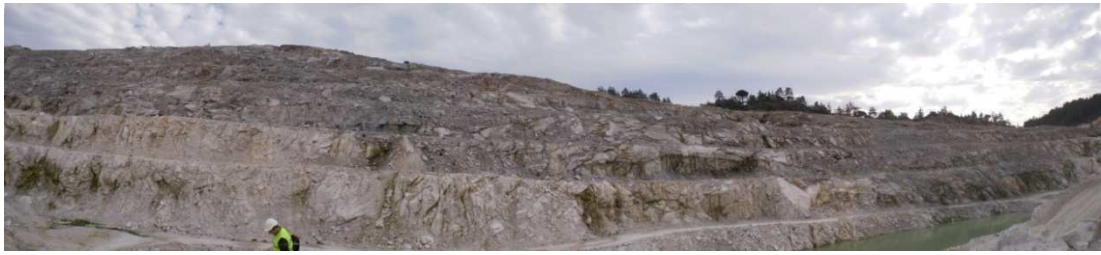
Figure 1.2 Panoramic view of the eastern slope of the Alipaşa open pit mine
