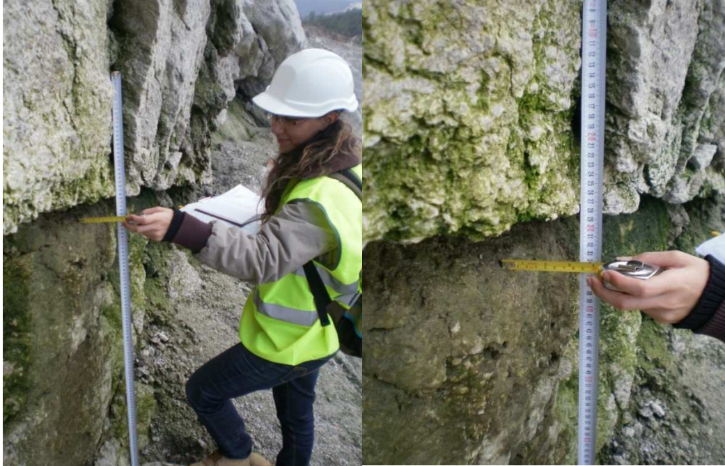
Figure 1.3 A shear displacement occurred on the foliation planes in the benches called as local planar slides.
