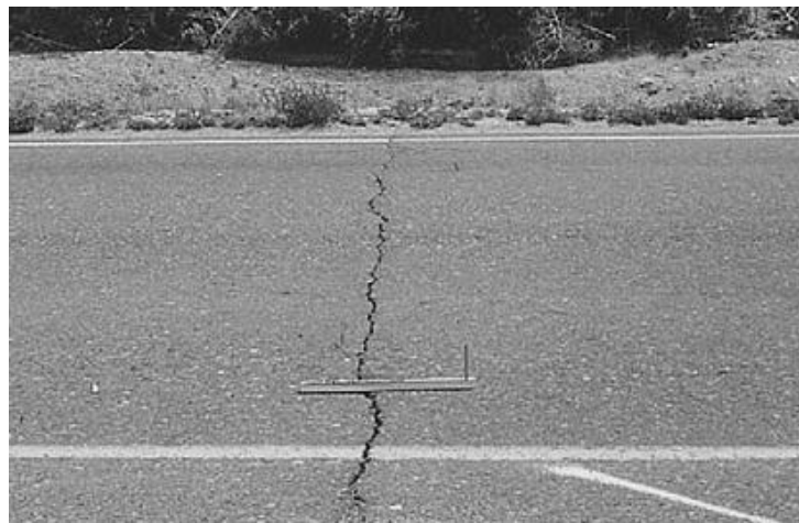
Figure 2.3 Thermal cracking (Fwa, 2006)
