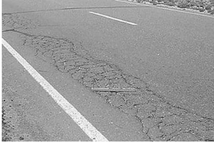
Figure 2.2 Advanced stage of fatigue cracking (Fwa, 2006)
