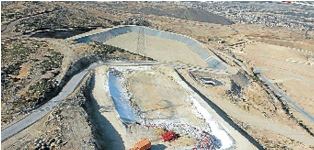
Fig 4.1 Harmandalı New Lot Construction
