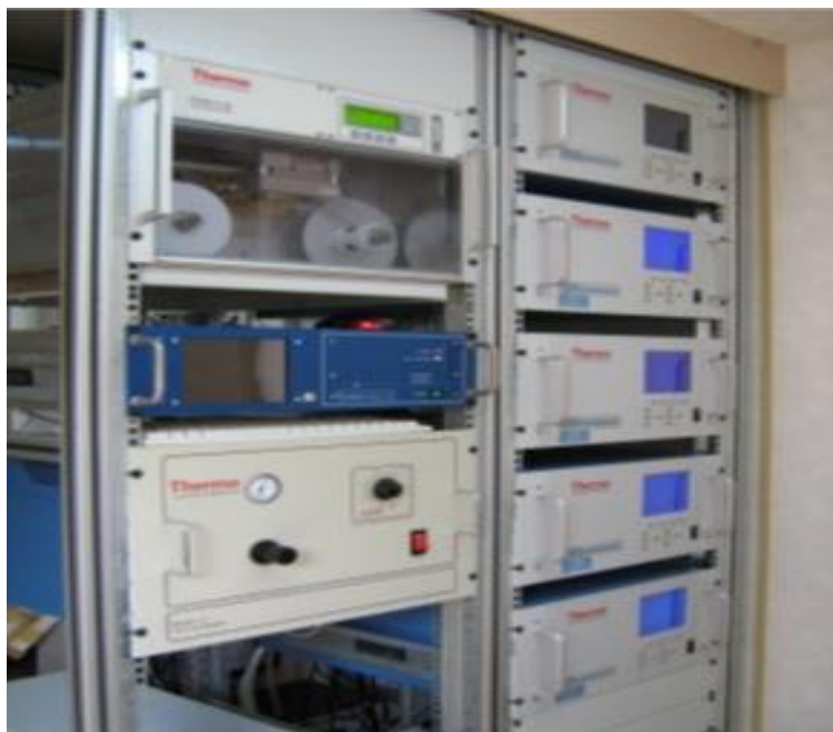
Figure 3.4 The interior of the mobile ambient air quality monitoring station owned by the Izmir Metropolitan Municipality.
