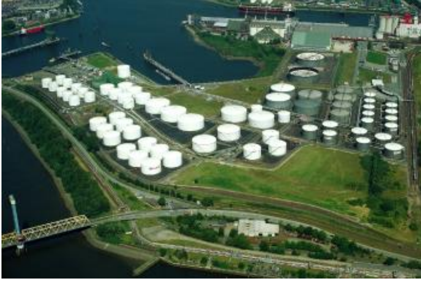
Şekil 29: OIL Tanking Hamburg terminali
