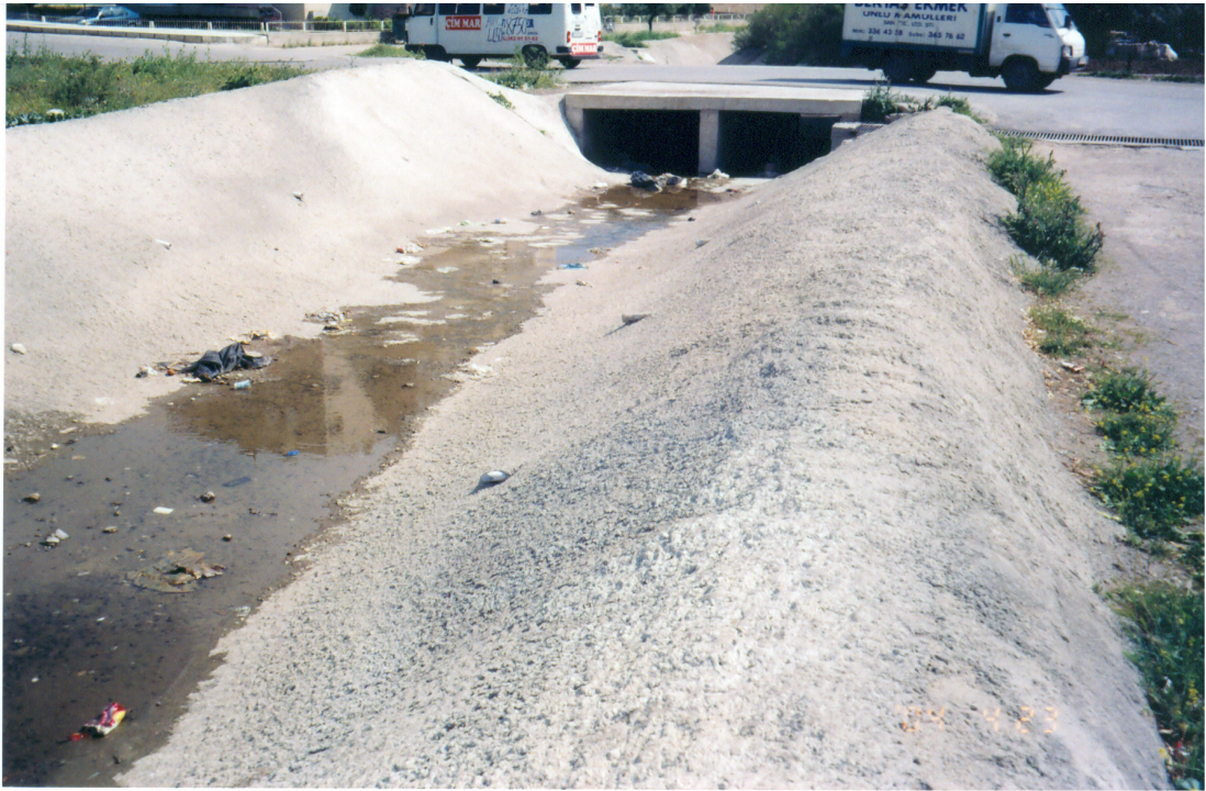
Figure A.25 Culvert on Kartalkaya River.
