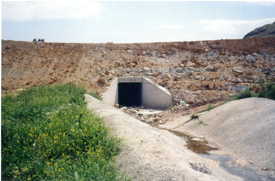
Figure A.24 Culvert on Kartalkaya River.
