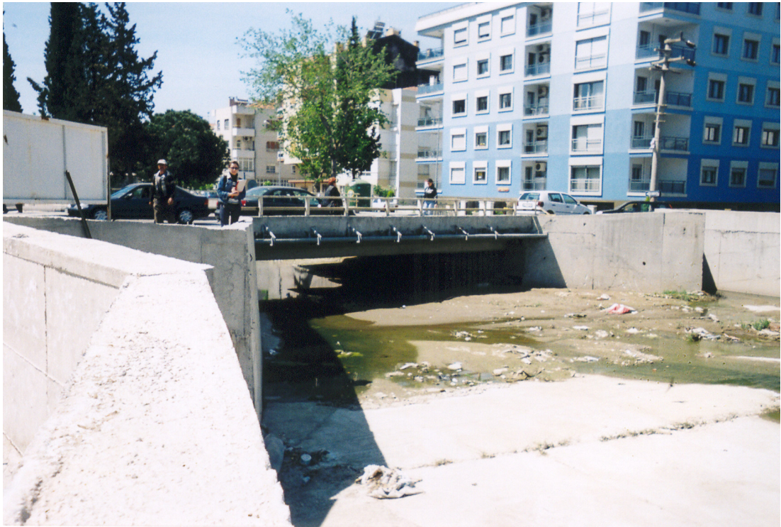
Figure A.17 Bridge on the main stream.
