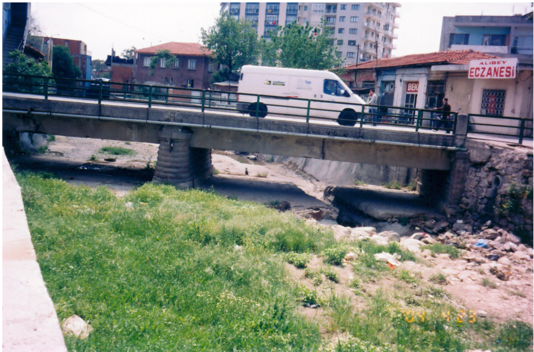
Figure A.20 Bridge on the main stream.
