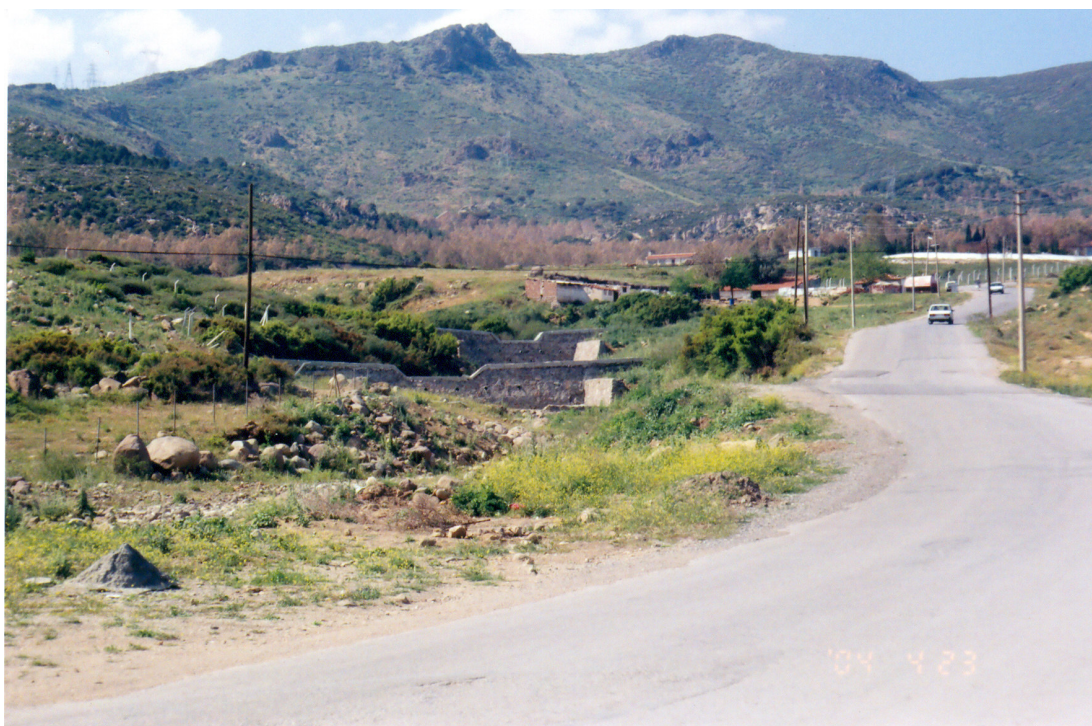
Figure A.31 Weirs on Koca River.
