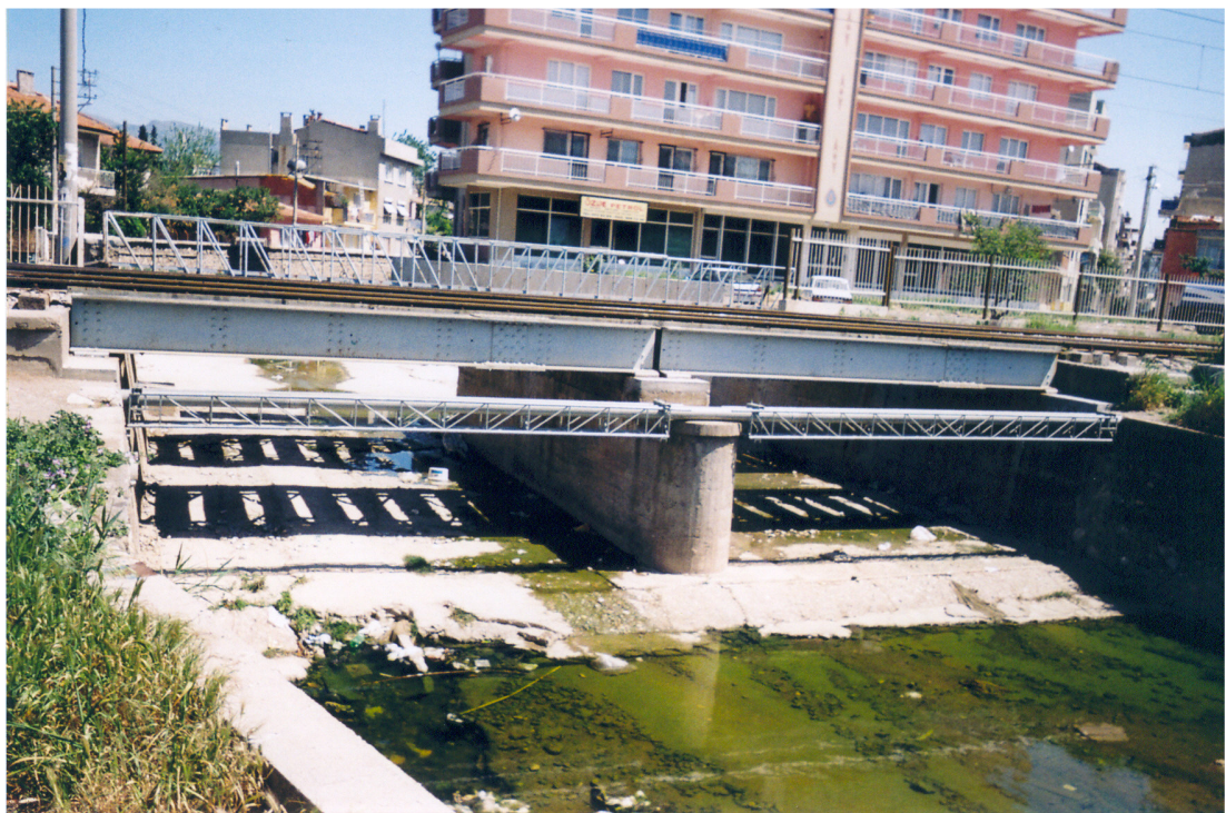
Figure A.18 Bridge on the main stream.
