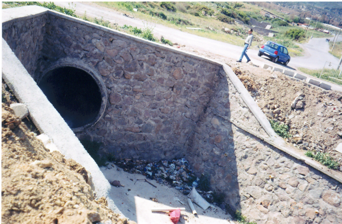
Figure A.30 Culvert on Koca River.
