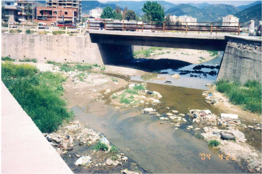
Figure A.21 Bridge on the junction.
