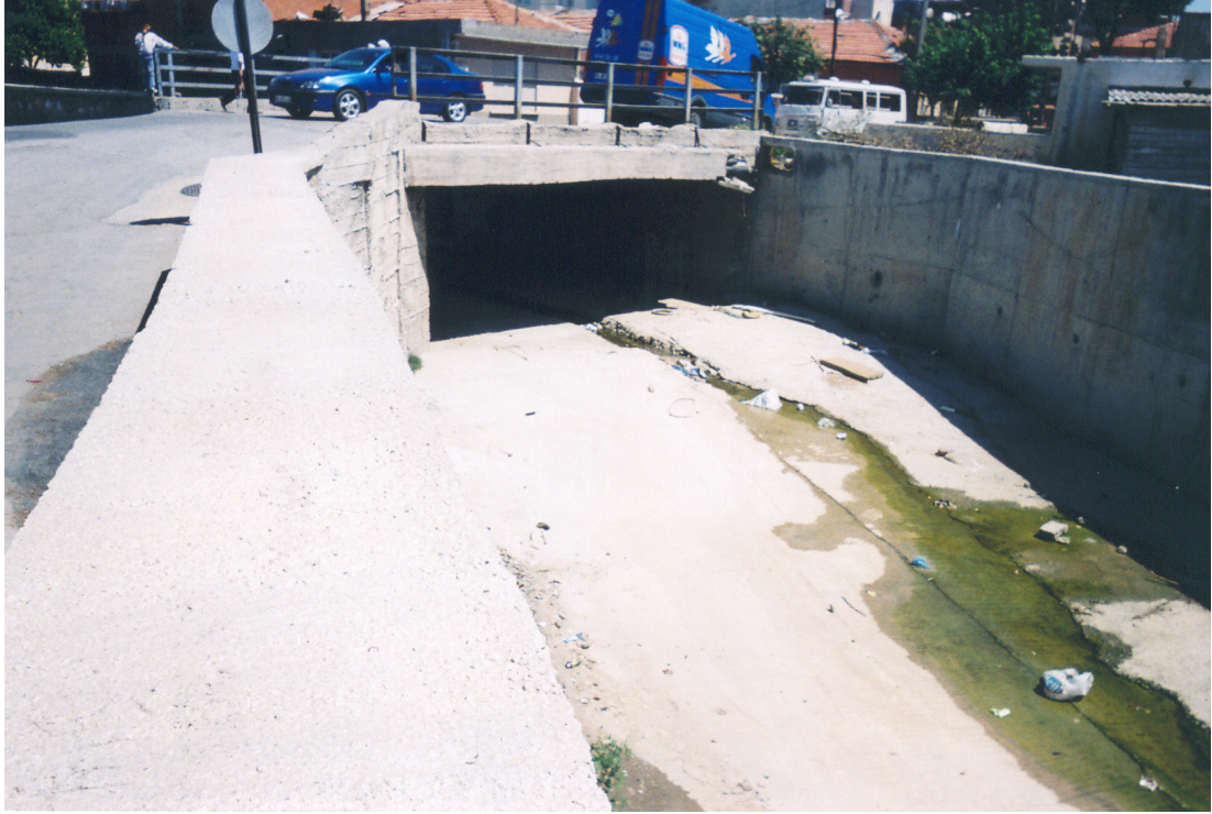
Figure A.19 Culvert on the main stream.
