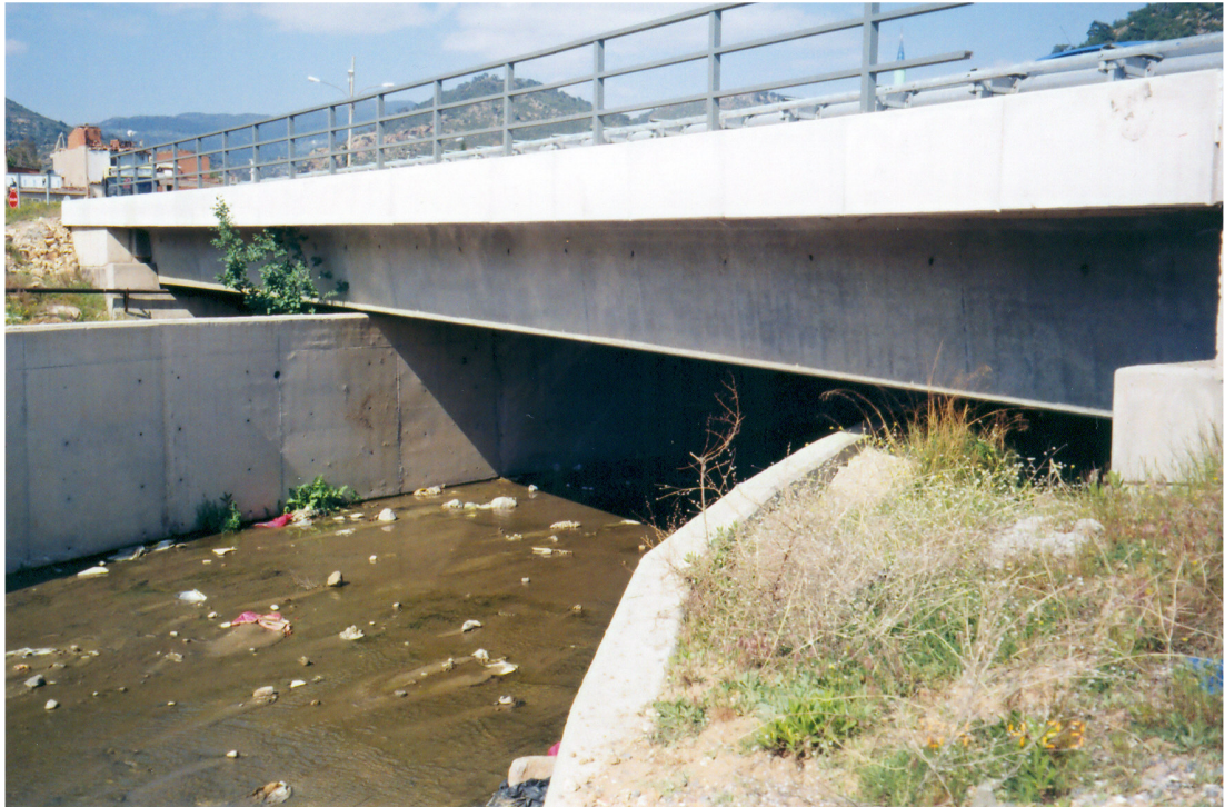
Figure A.29 Bridge on the main stream.
