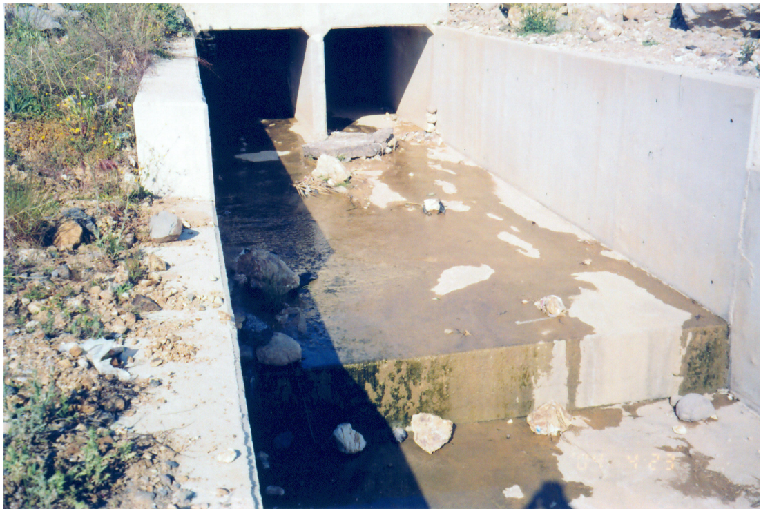
Figure A.28 Culvert on Eskisekikoy River.
