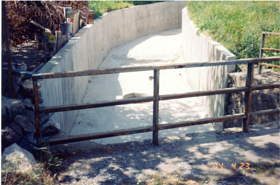
Figure A.23 Back view of a bridge on Kartalkaya River.
