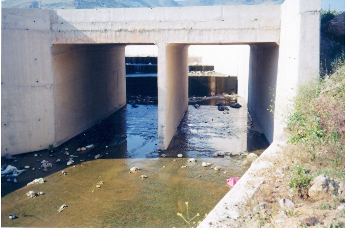
Figure A.27 Culvert on Eskisekikoy River.
