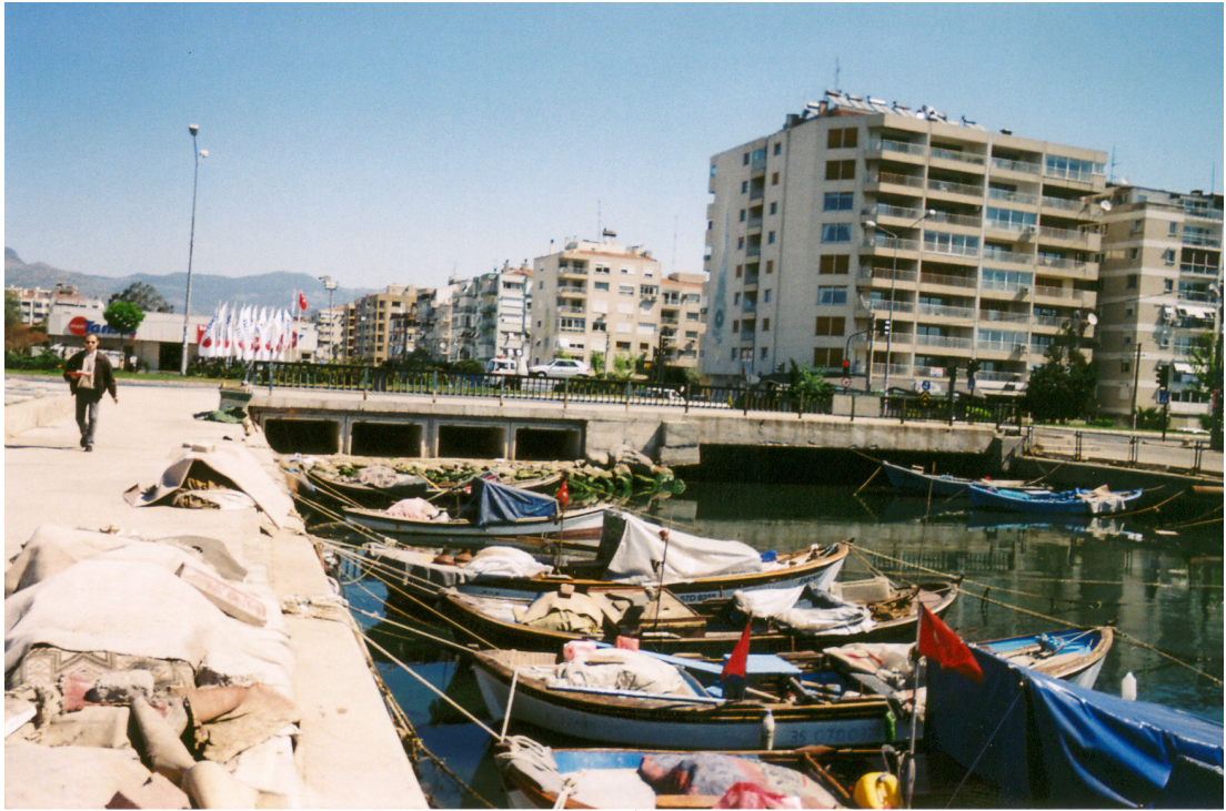
Figure A.15 Front view from the outlet.
