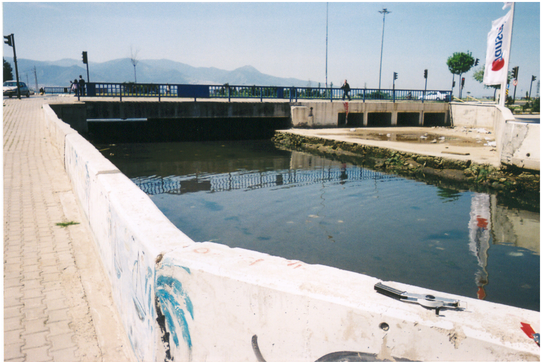
Figure A.16 Back view from the outlet.
