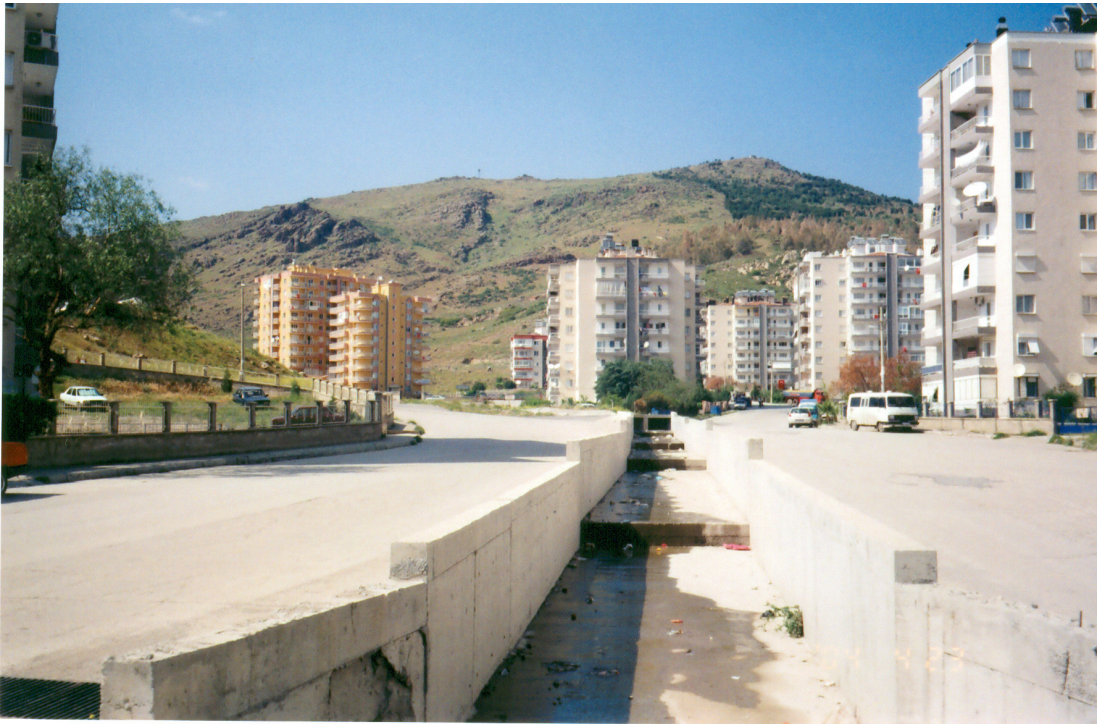
Figure A.26 Culvert and on Kartalkaya River.
