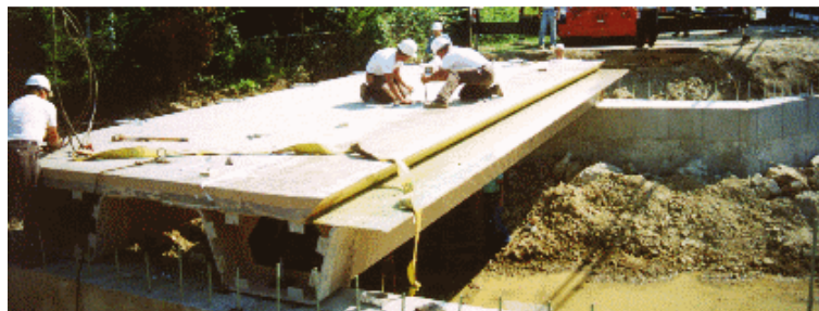
Figure 2.23 An epoxy/glass fiber-reinforced construction of a bridge. ( www.bceo.org , 2008)
